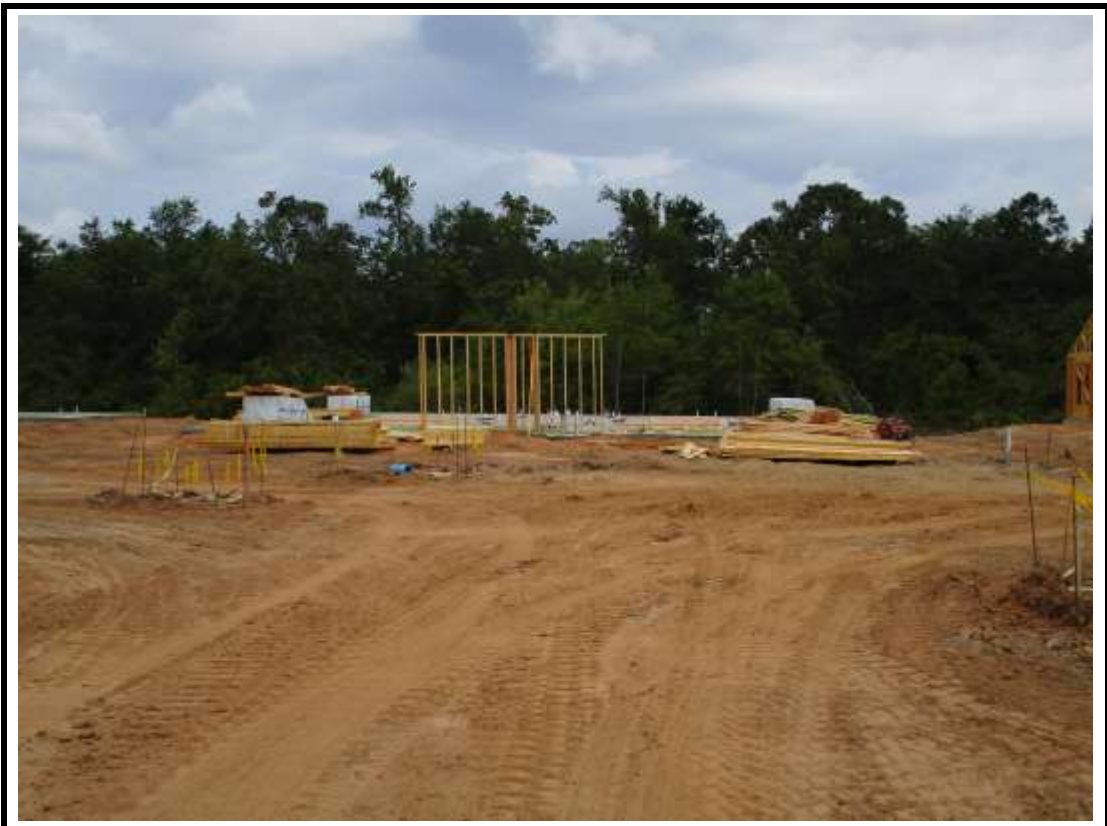
Photograph 7: Building 9 framing started.
