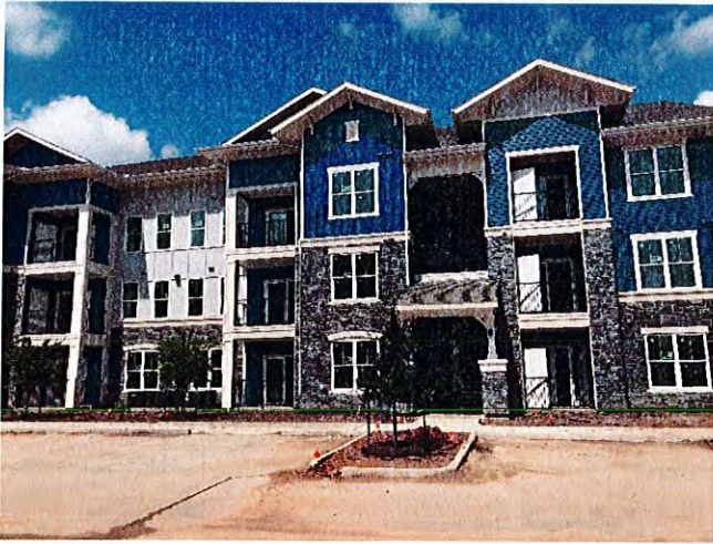
Overall view of building 3.
