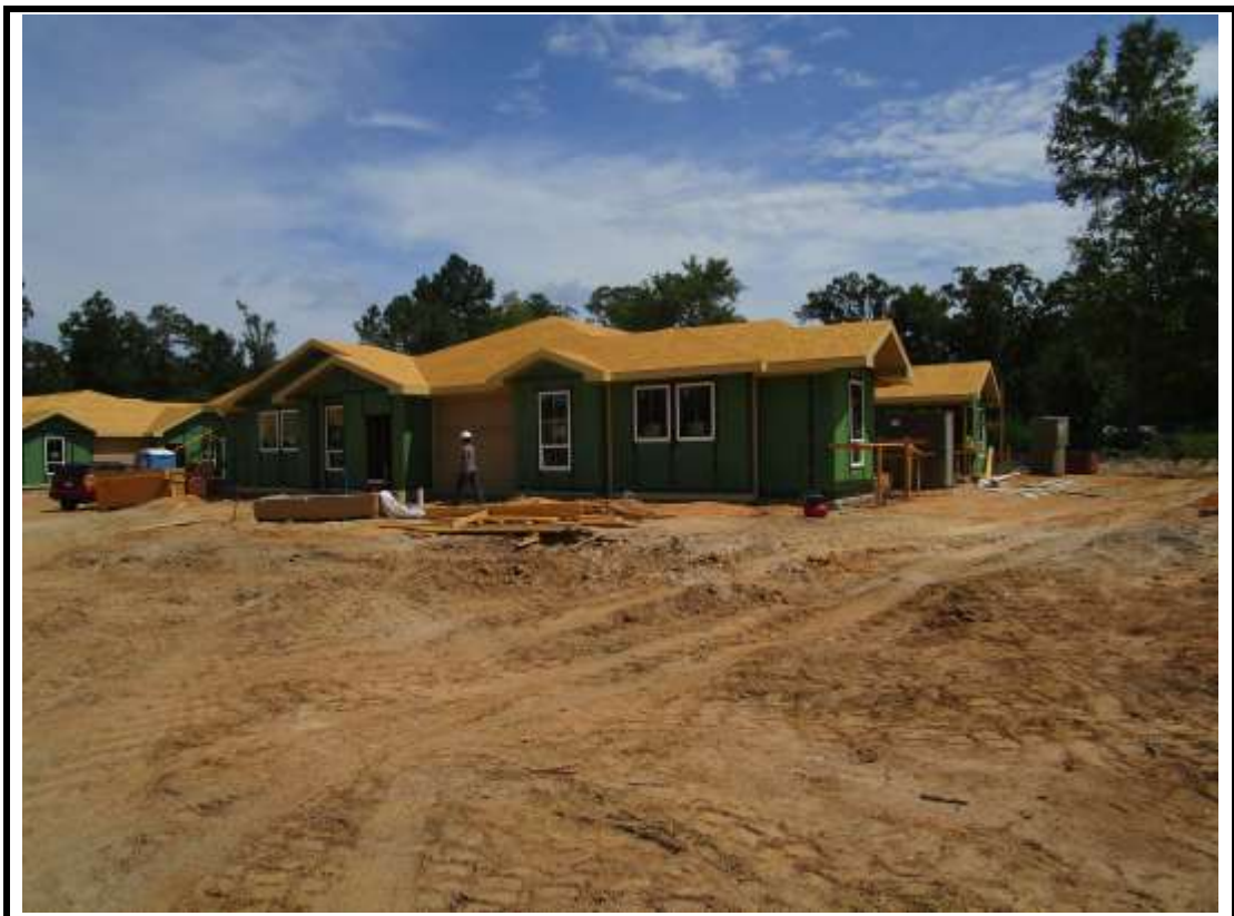
Photograph 8: Building 8 roof and wall sheathing complete.
