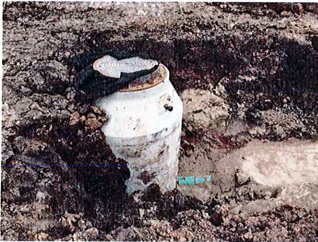
The manholes have been installed throughout the site.
