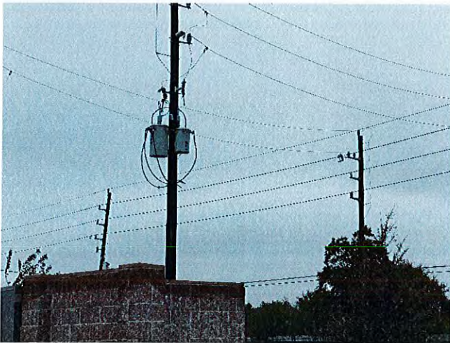
View of the new electrical transformers that had to be installed.
