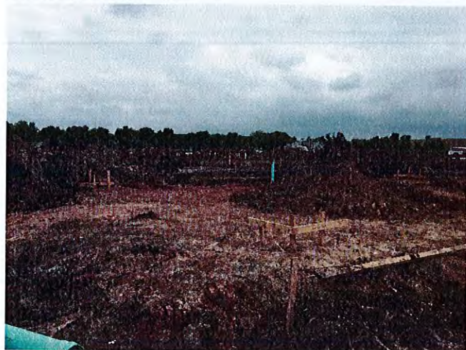
Surveying and staking is underway at the clubhouse.
