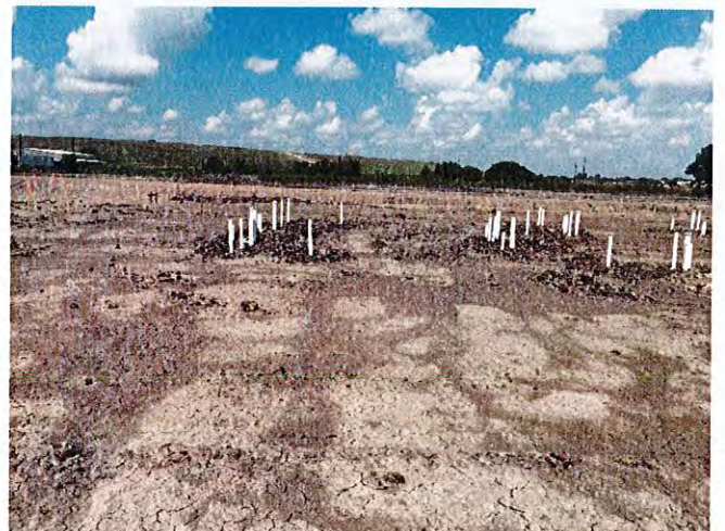
Underground utilities are substantially complete at building #4.
