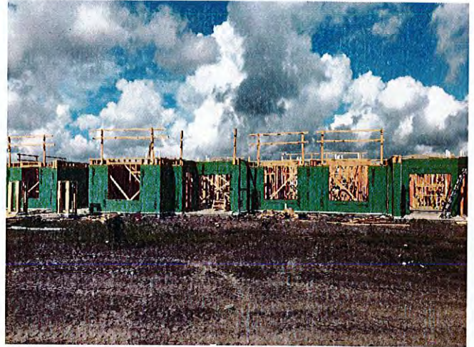
Overall view of Building 2.
