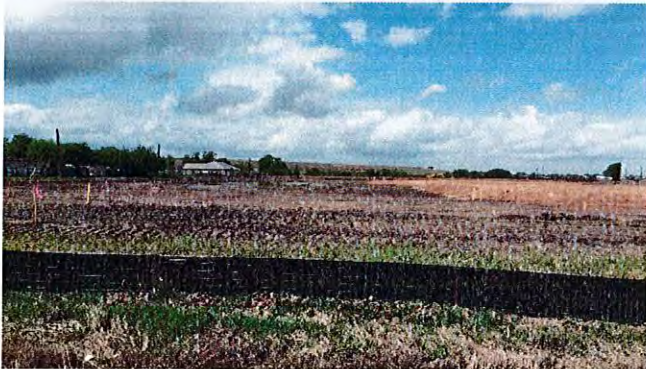
Select fill and compaction at building pad #4.
