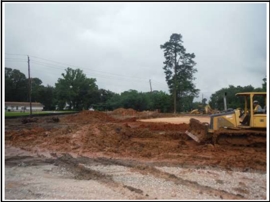
Photograph 1: Site work at entrance.
