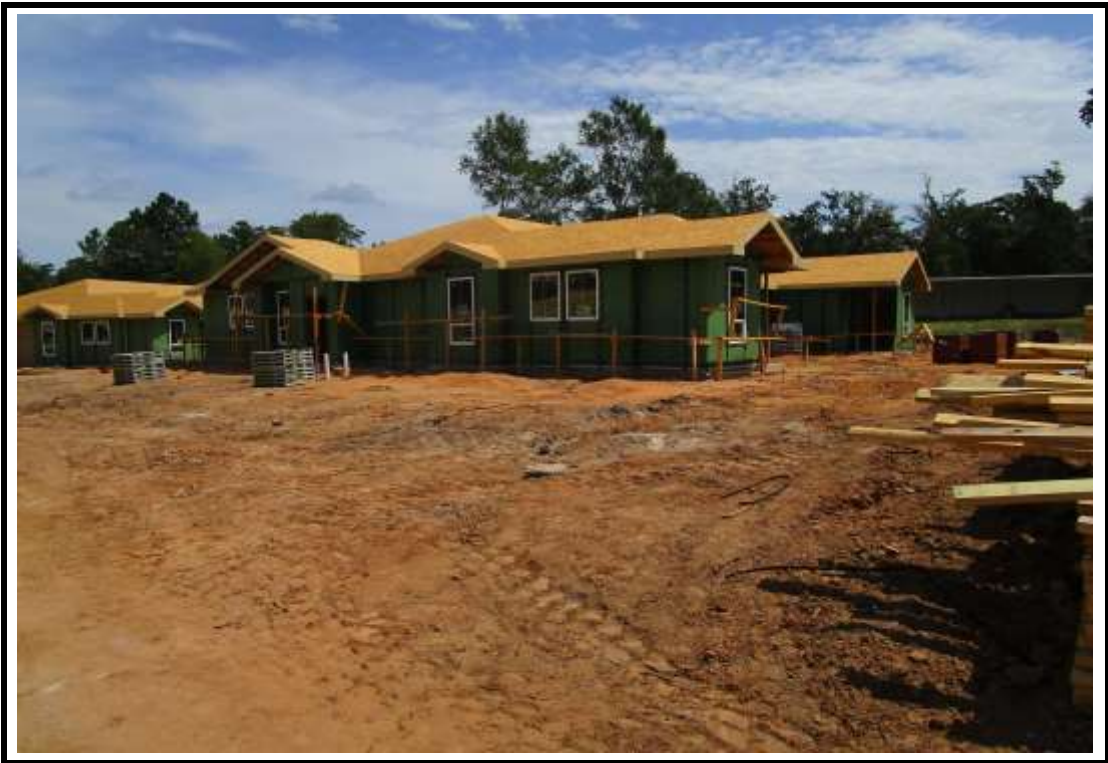
Photograph 6: Building 6 roof sheathing.
