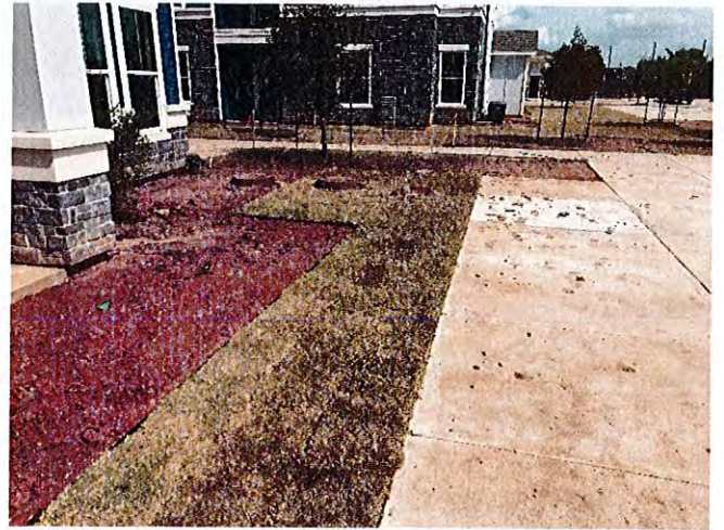
Landscaping was being placed around the clubhouse.
