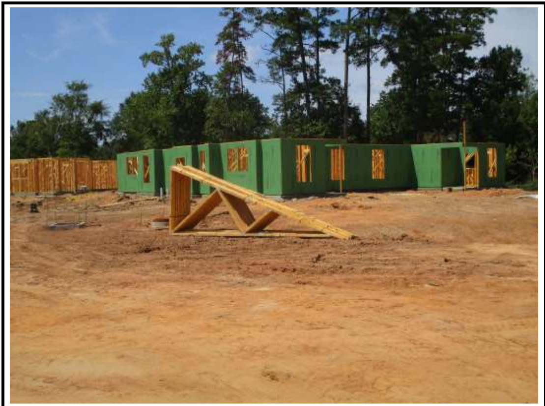
Photograph 15: Pad site building 17 framing & sheathing.
