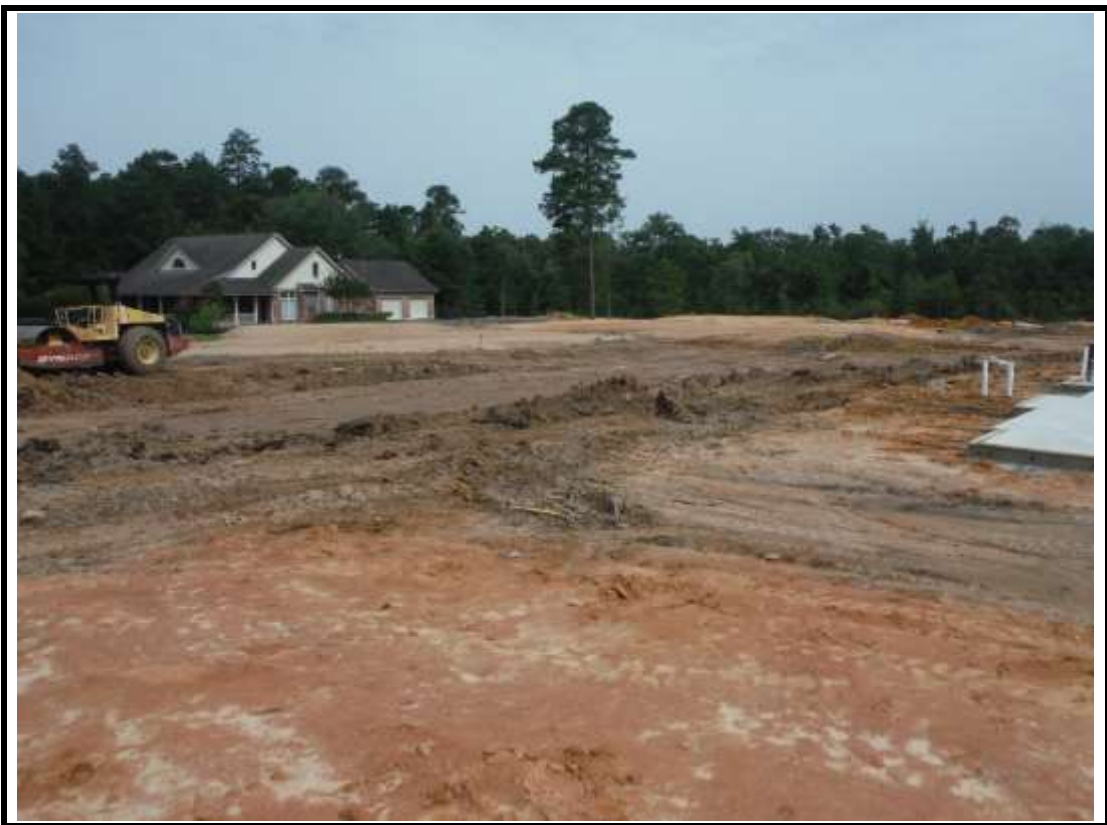
Photograph 4: Street grading in progress.
