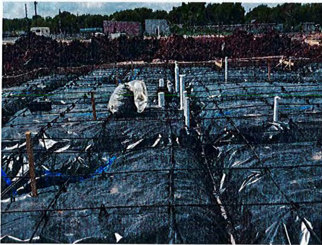
The formwork and vapor barrier are complete at the clubhouse.
