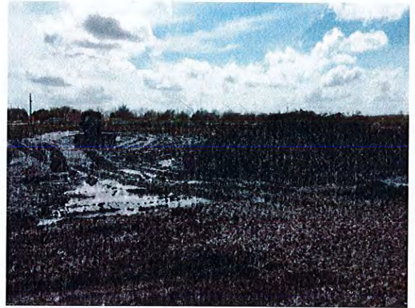
2. The bull dozer is removing excess water from the site.
