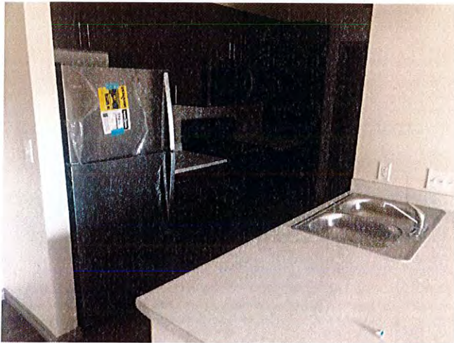
Appliances, countertops and cabinets were in place throughout building 1.
