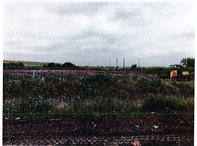
Overall view of the cricket field which had earthwork nearing completion.
