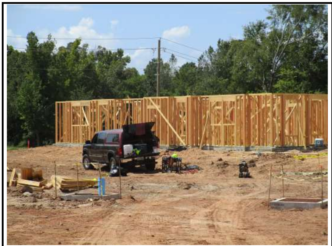
Photograph 16: Building 18 framing progress.
