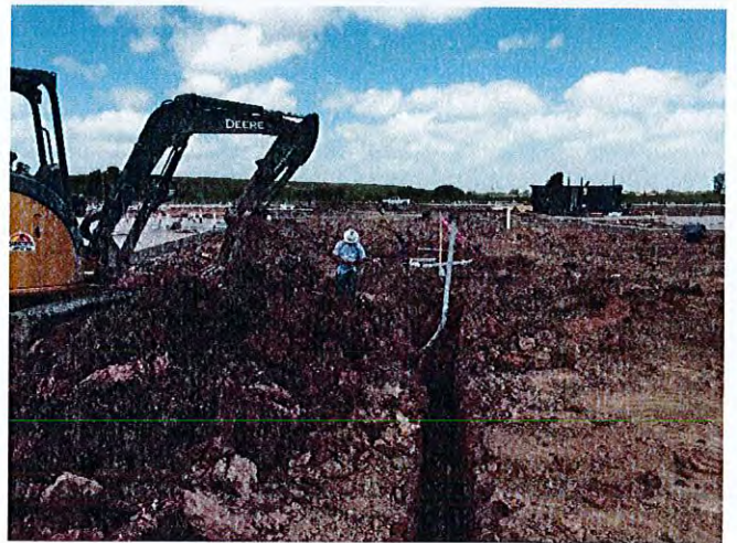
Electrical conduit was being buried at building 4.
