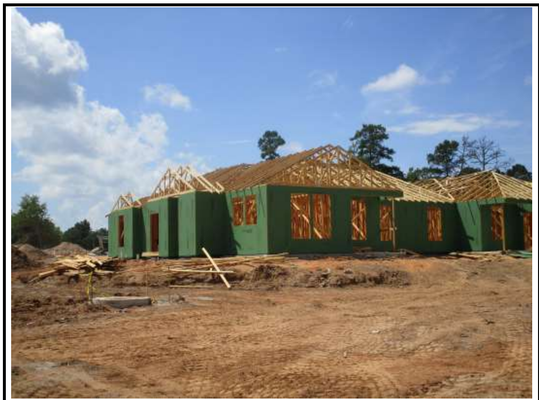
Photograph 12: Building 11 roof trusses in progress.
