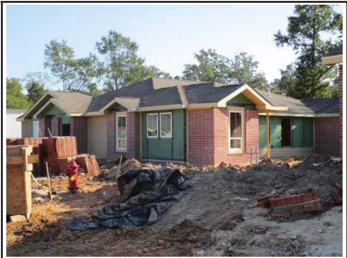
Photograph 7: Building 6 ready for siding.
