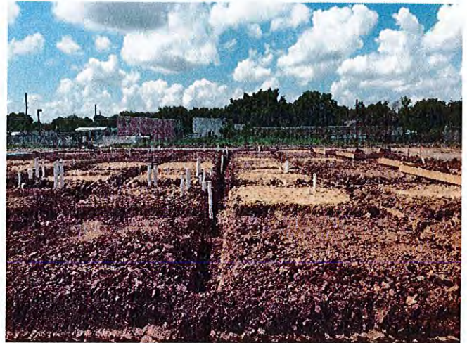
Excavation for the grade beams at building 2 is underway.
