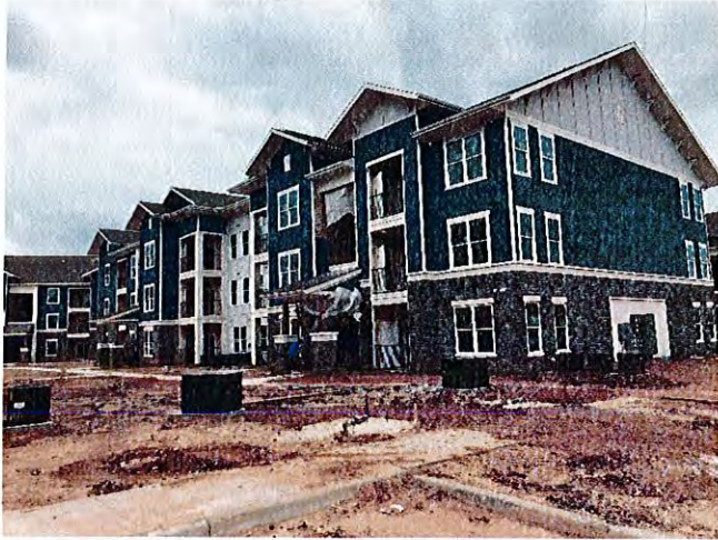
Overall view of building 3 with siding and painting operations substantially complete.
