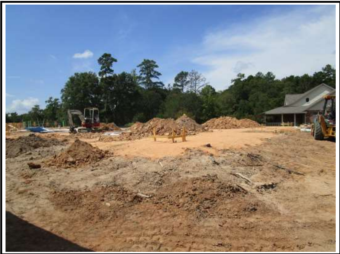
Photograph 13: Building 13 pad site with underground plumbing in progress.
