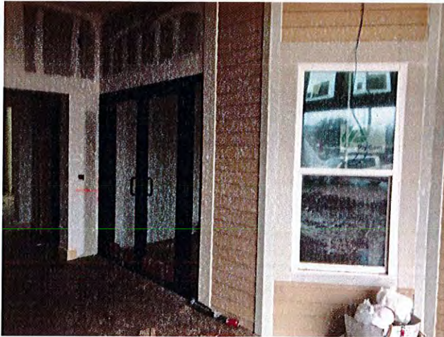
Interior doors and windows were being installed.
