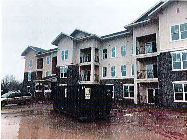
Overall view of Building #1.
