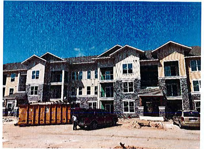
Overall view of building 4.
