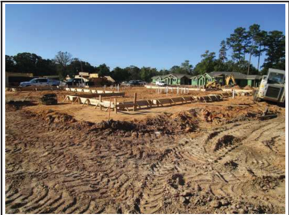
Photograph 13: Building 13 formed for foundation.
