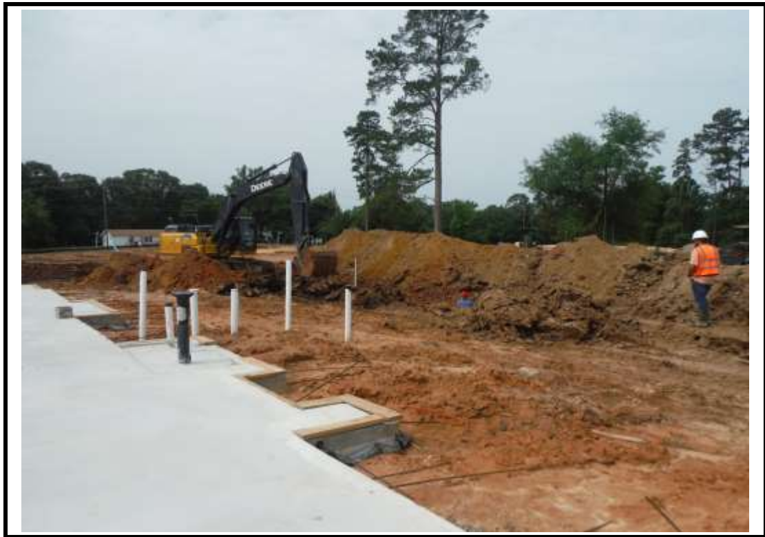
Photograph 5: Underground utility excavation.
