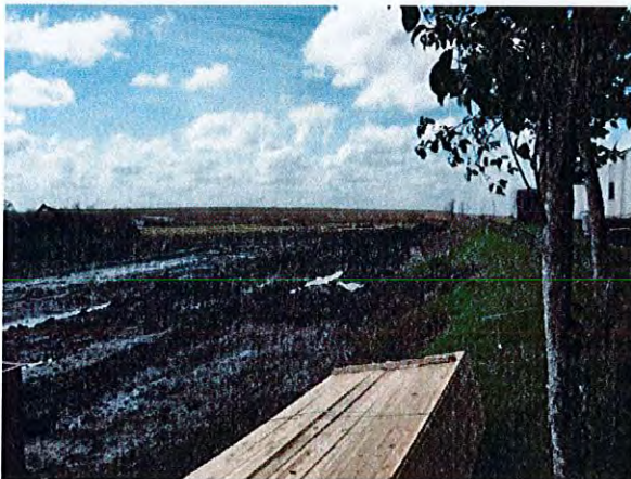
3. The site has been grubbed.
