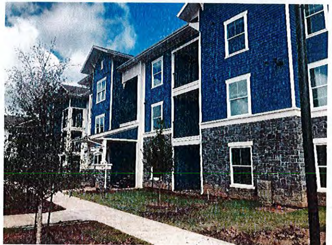
Overall view of building 1 with exterior work complete.
