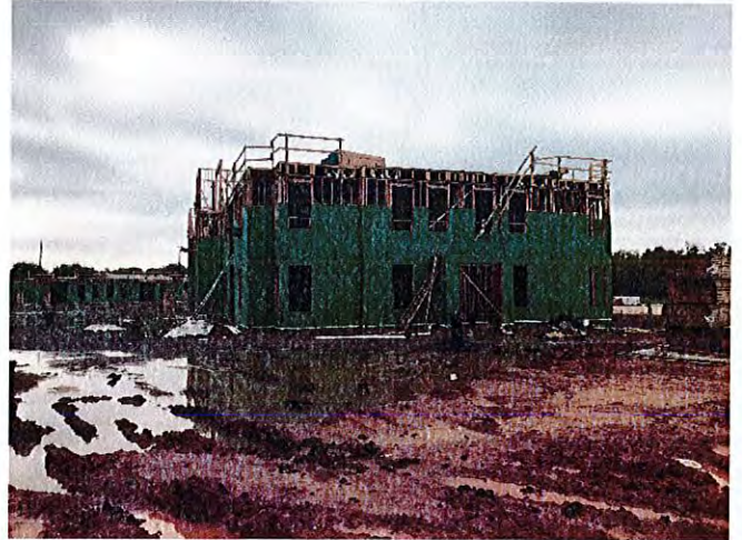
Overall view of building 5.
