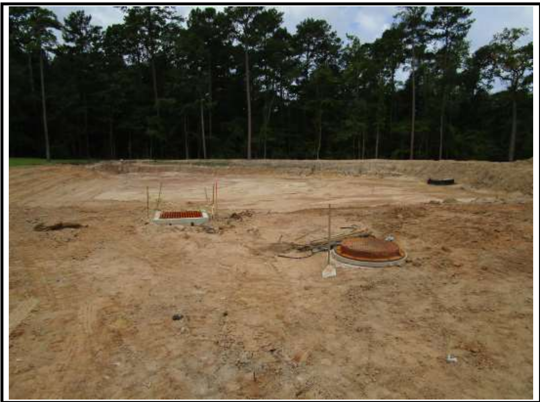
Photograph 8: Detention pond complete.
