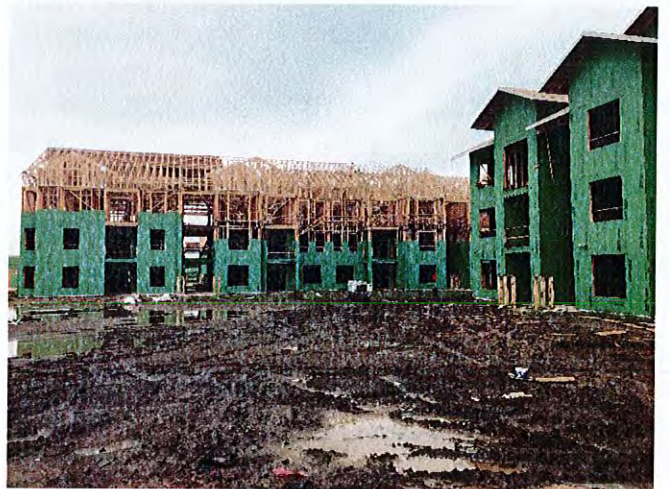
Roof trusses were being installed on building 2.
