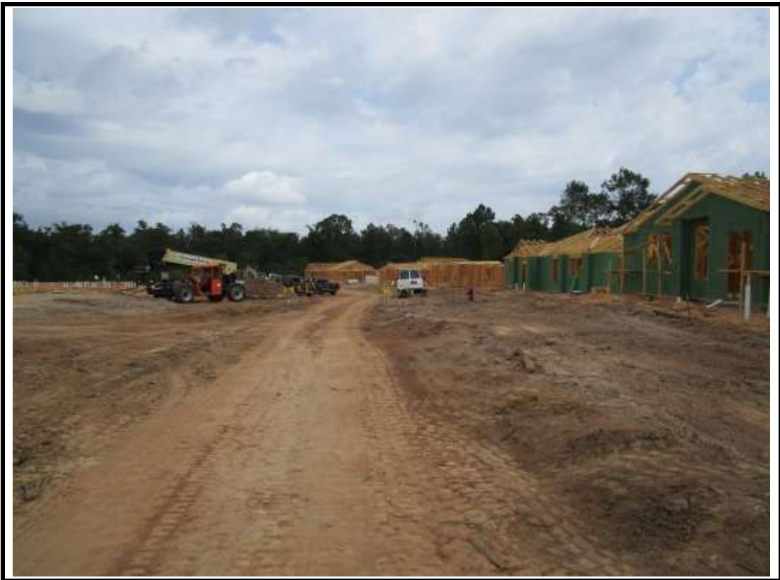
Photograph 4: Street grading in progress, in front of buildings 4 through 7.
