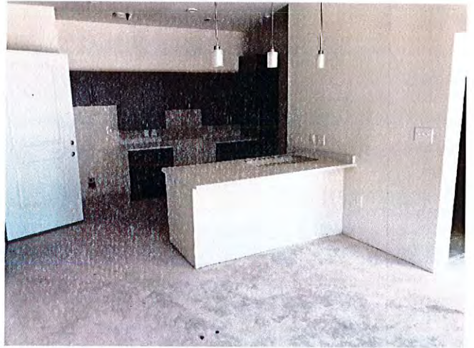
Overall view of the kitchen in building 3.
