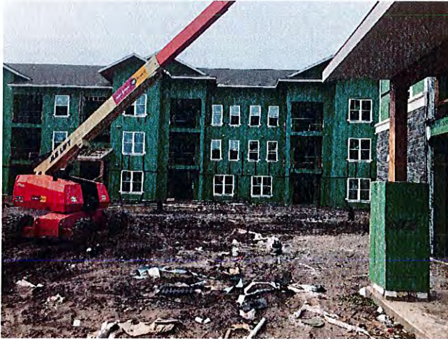
Overall view of Building 2.
