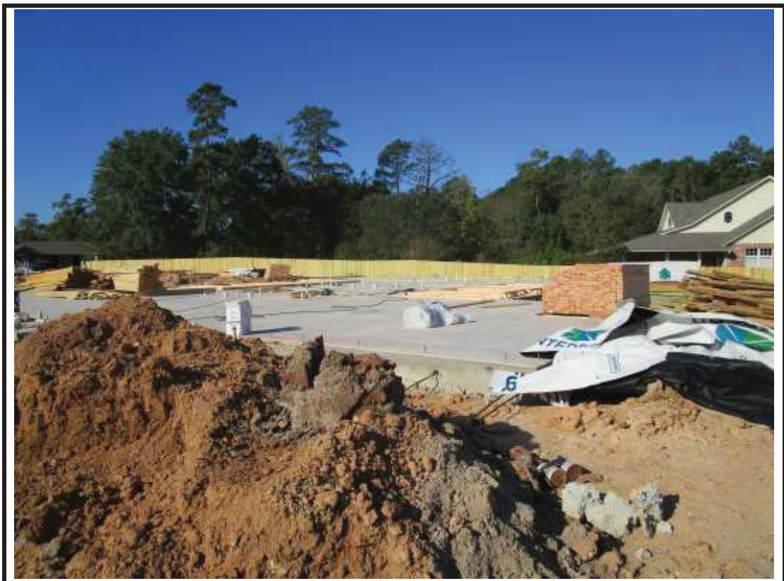
Photograph 12: Building 12 Foundation poured.
