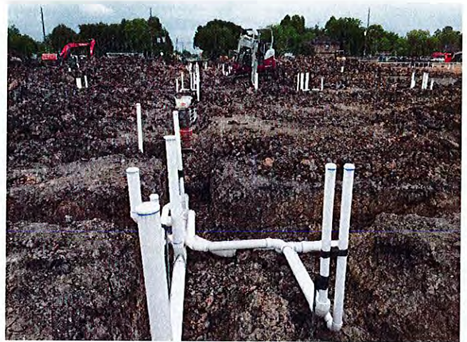
Underground utilities are underway at building 1.
