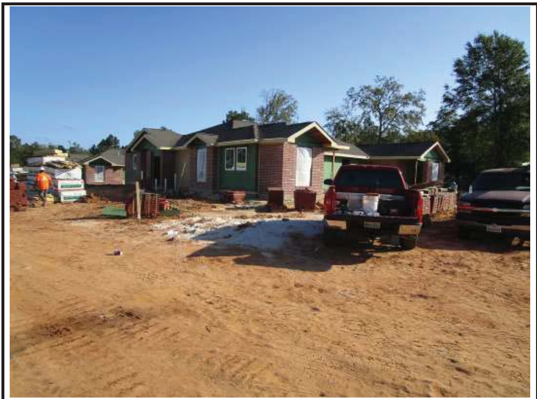
Photograph 4: Building 4 exterior progress.
