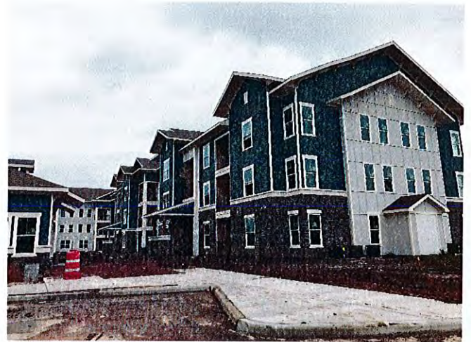
Building 1 had exterior work substantially complete.
