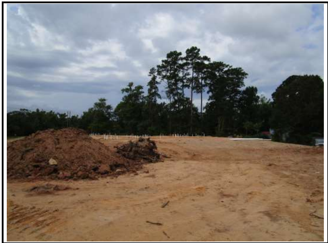
Photograph 14: Drive between buildings 15 and clubhouse grading.
