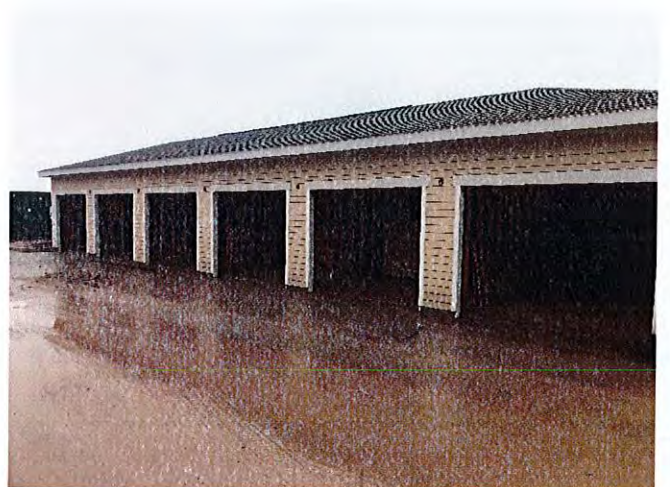
The exterior parking garages were nearing completion.
