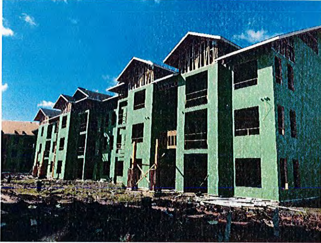
Overall view of building 2.
