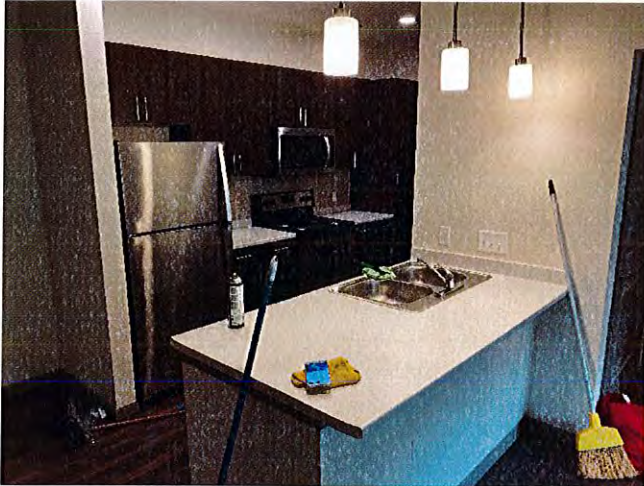
Final cleaning operations were nearing completion at unit 3401.
