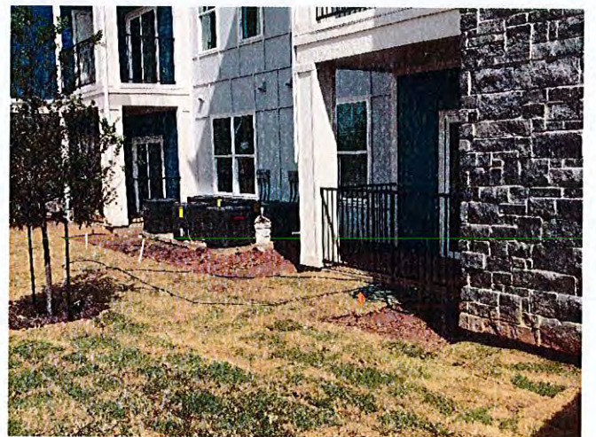
Trees and grass in place at building 1.
