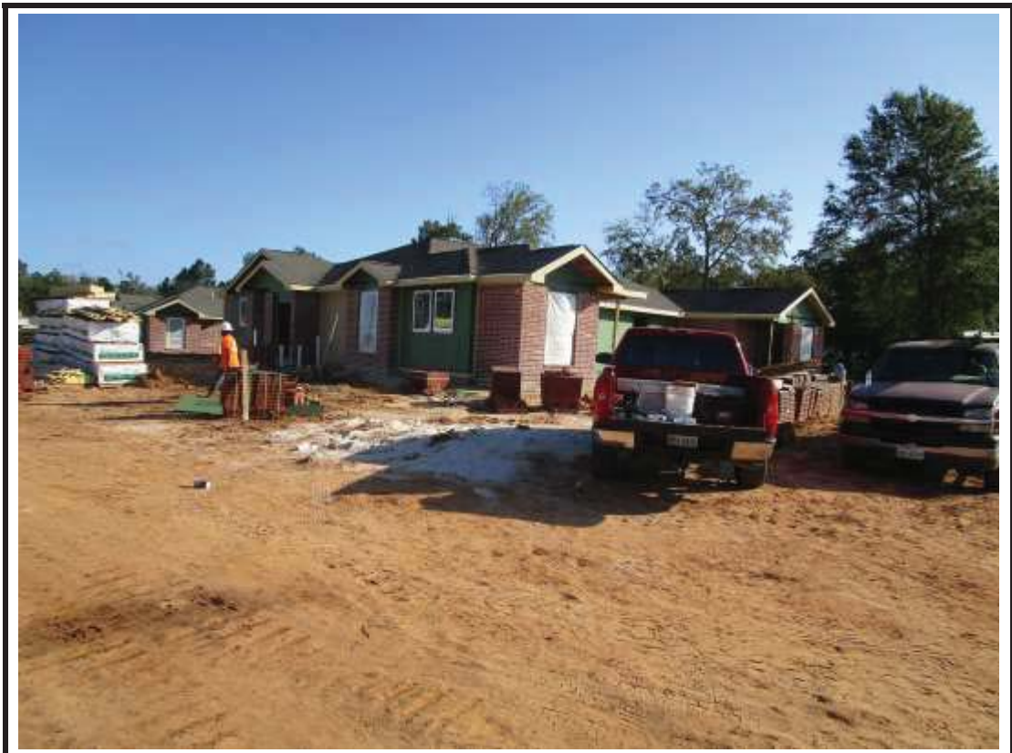
Photograph 3: Building 3 exterior brick installed.
