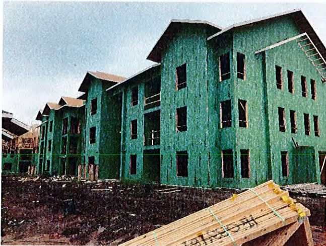
View of building 1 weatherproofing operations were well underway.
