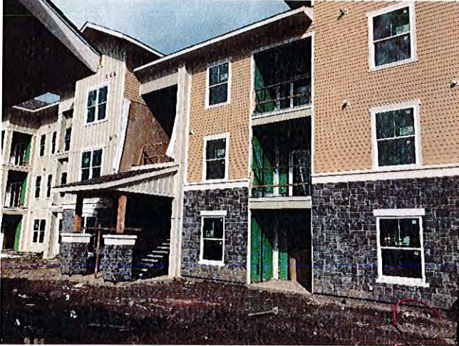
Overall view of Building #1.
