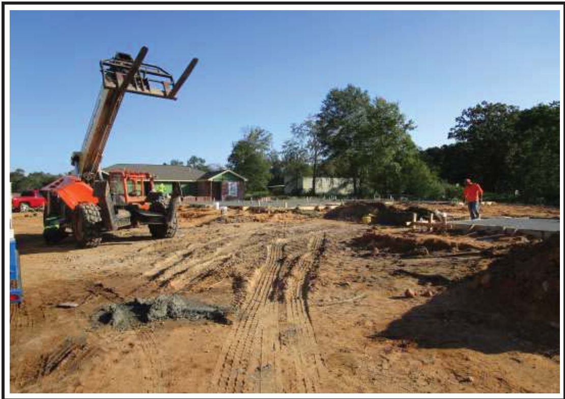
Photograph 2: Building 2 foundation poured.
