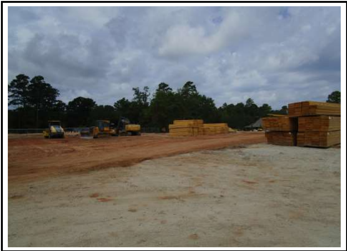
Photograph 1: Large quantities of lumber on site for framing.
