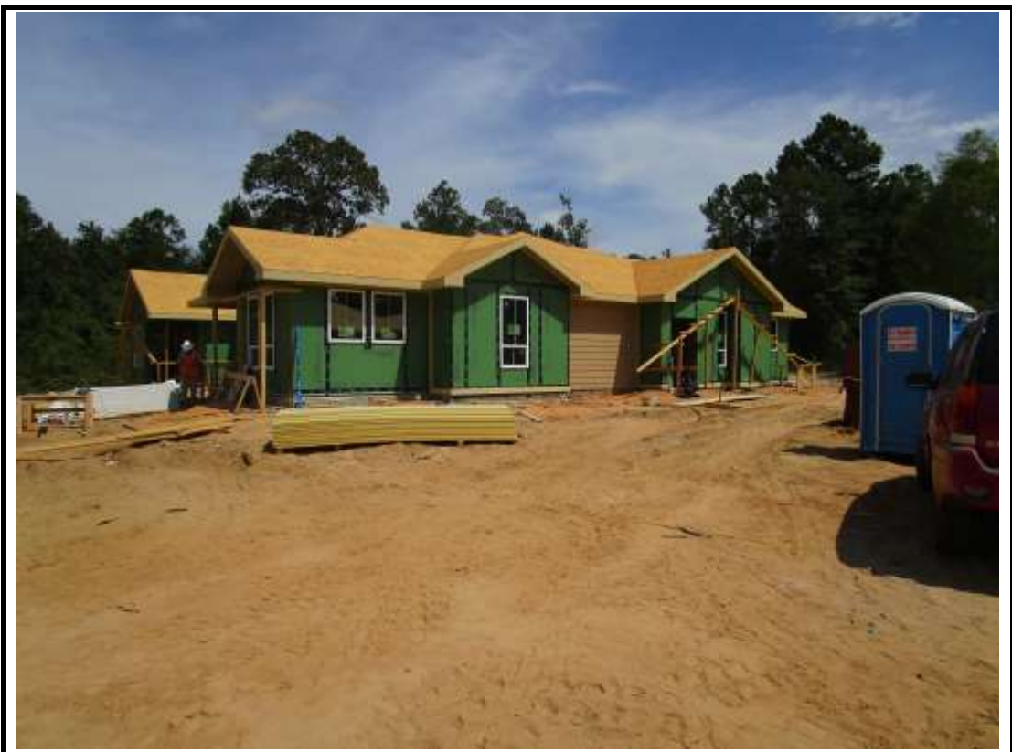
Photograph 10: Building 8 siding started.
