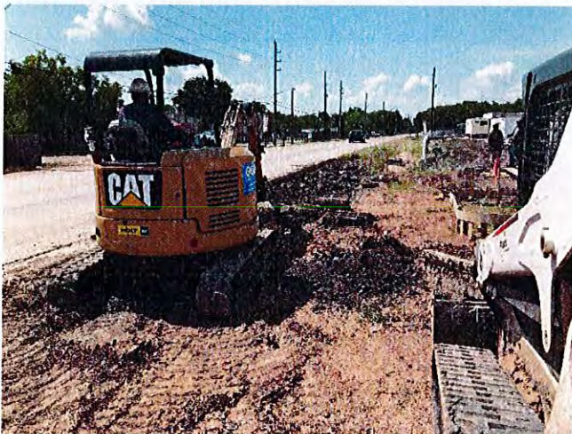
Preparation for tie-in work for the approaches is in progress.
