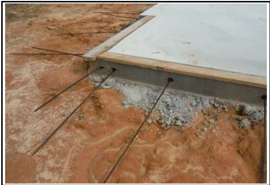
Photograph 6: Building 4 foundation stabilizers.
