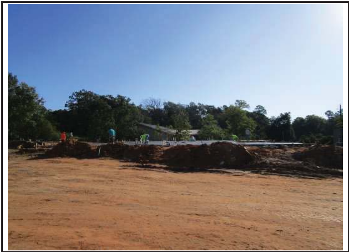
Photograph 1: Building 1 foundation being poured.
