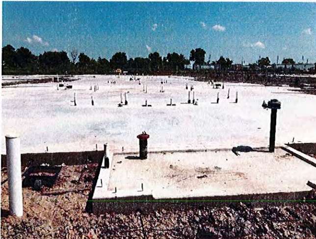
Overall view of Building 3 slab.
