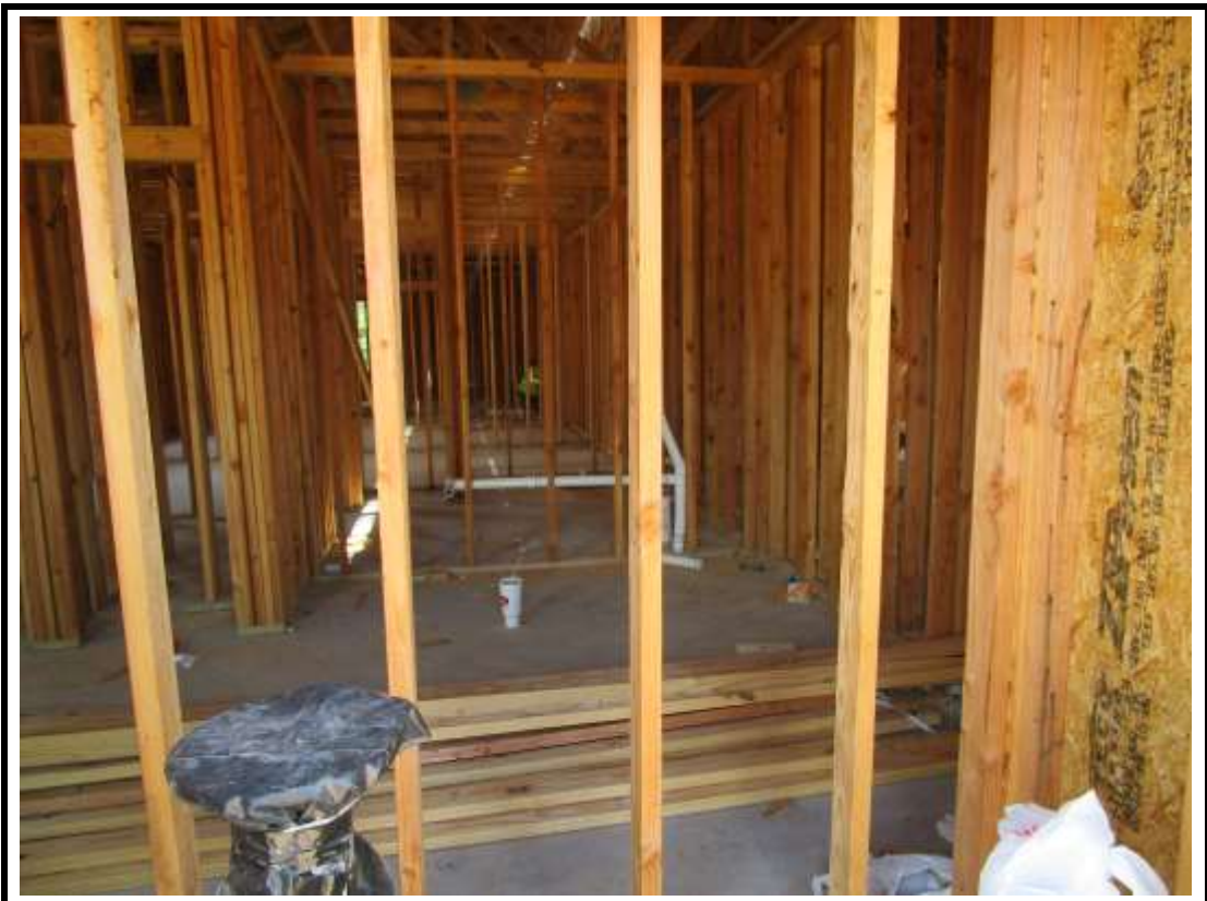
Photograph 9: Building 8 plumbing rough in.
