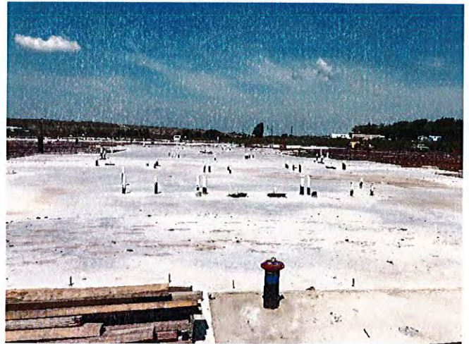
Overall view of Building 2 slab.
