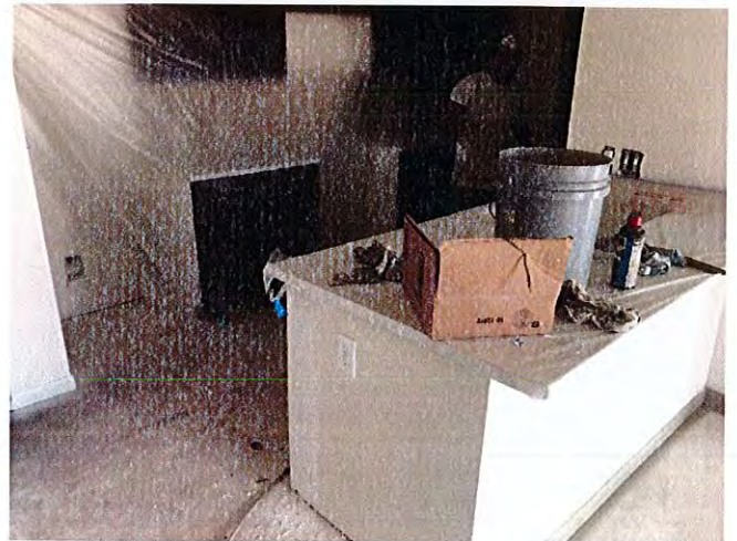
Caulk work was on-going, cabinets and countertops had been installed.
