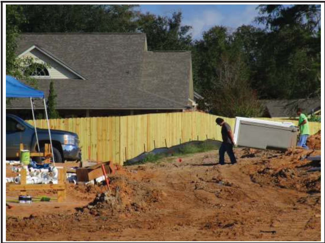
Photograph 15: Privacy fence installed next to neighboring home.
