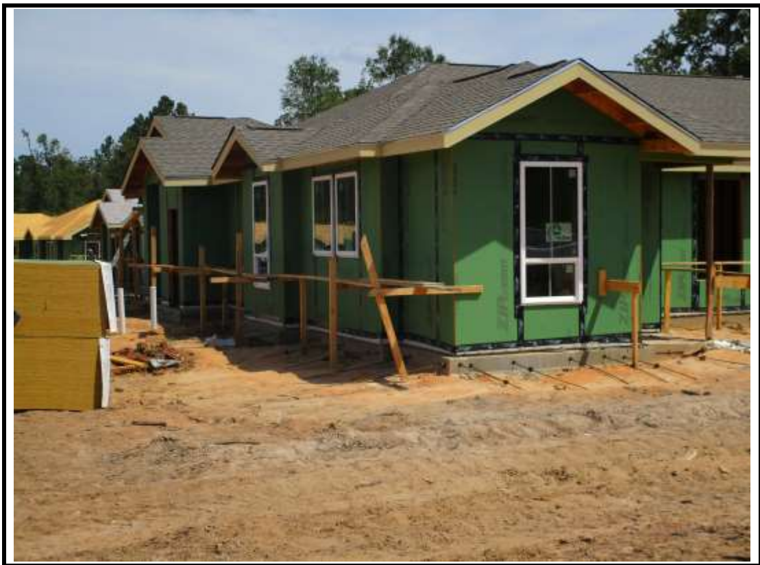
Photograph 4: Building 4 roof and wall sheathing complete.
