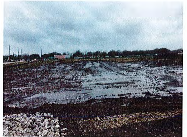
6. Northern portion of the site that has been cleared and grubbed.
