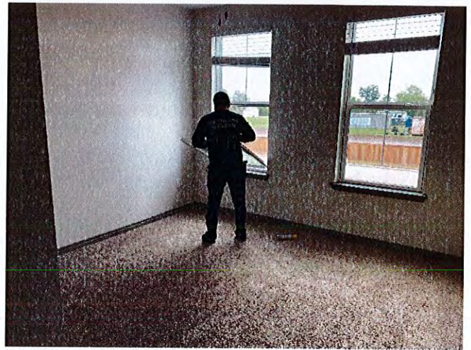
Final touch up work was nearing completion.
