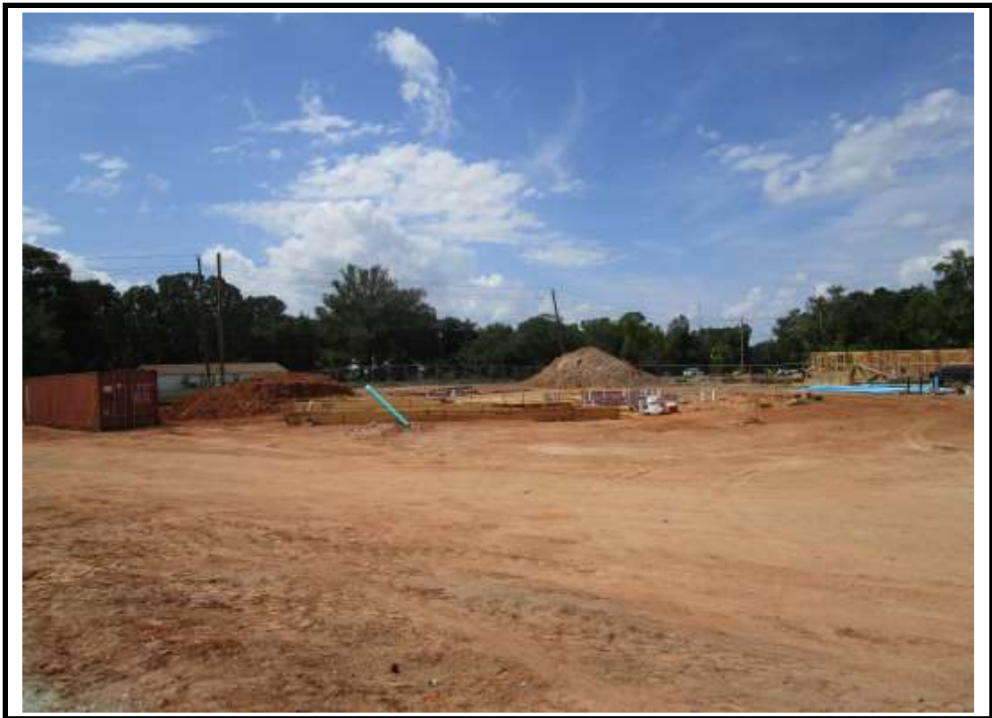
Photograph 1: Clubhouse pad plumbing rough in.
