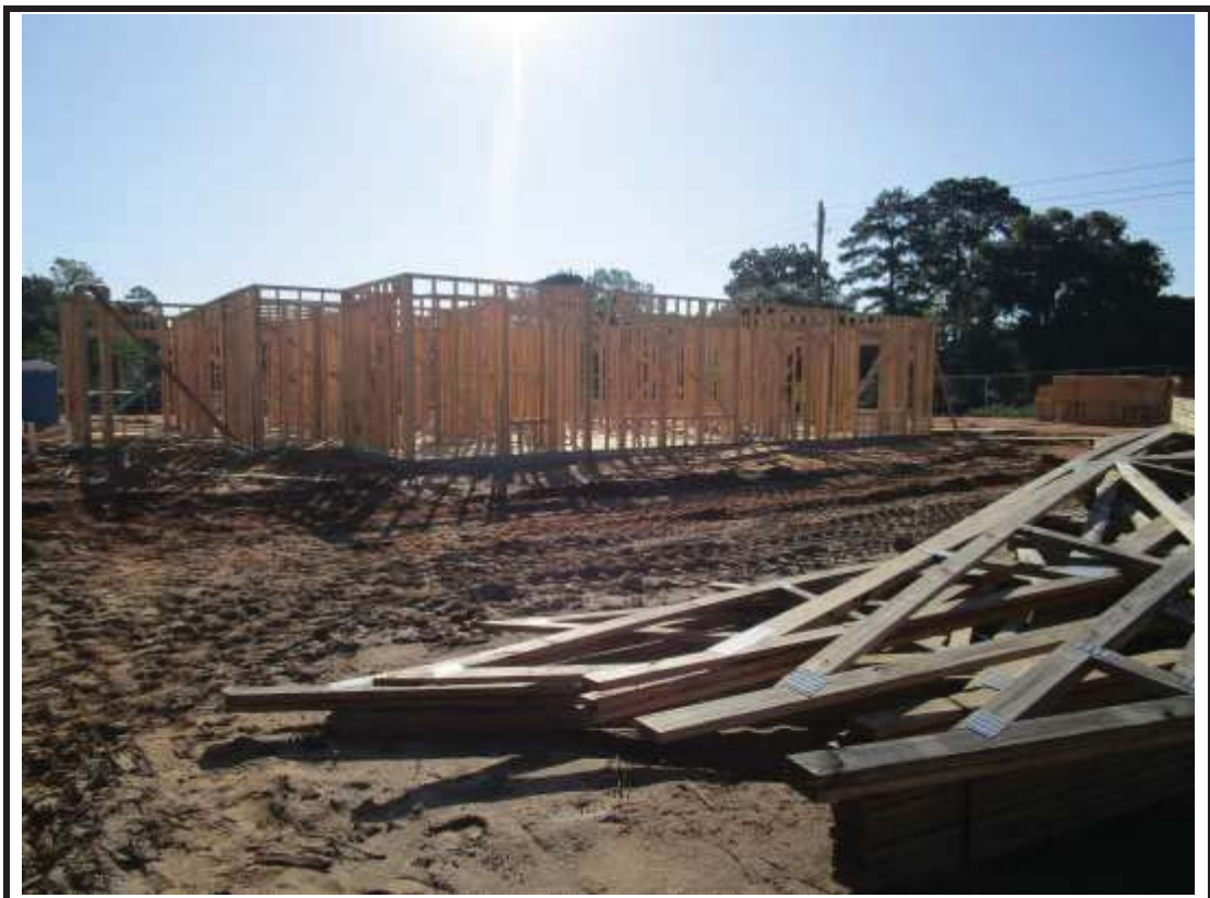
Photograph 14: Clubhouse framing in progress.
