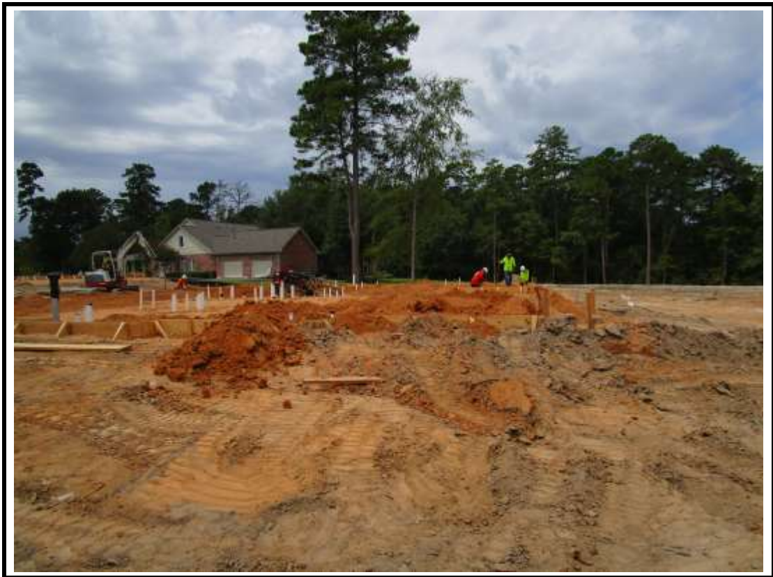
Photograph 9: Building 1 pad ready for concrete pour.
