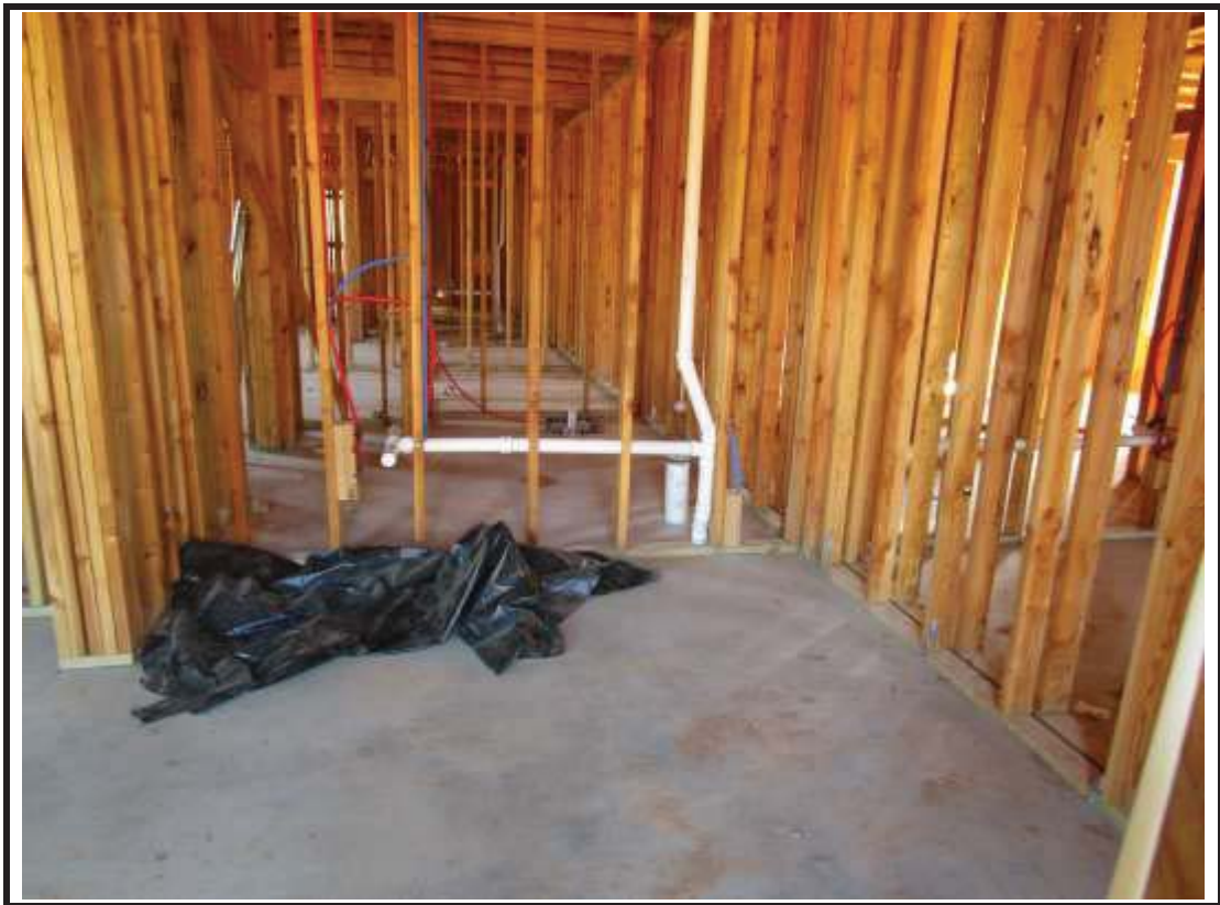
Photograph 10: Building 10 plumbing rough in.
