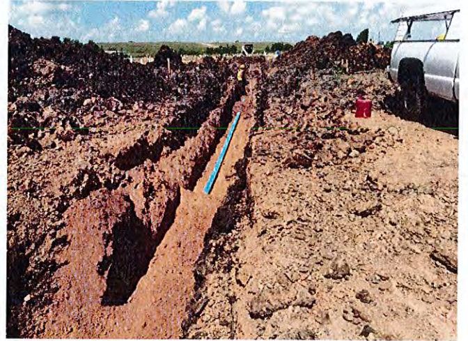
The underground fire line was being backfilled.
