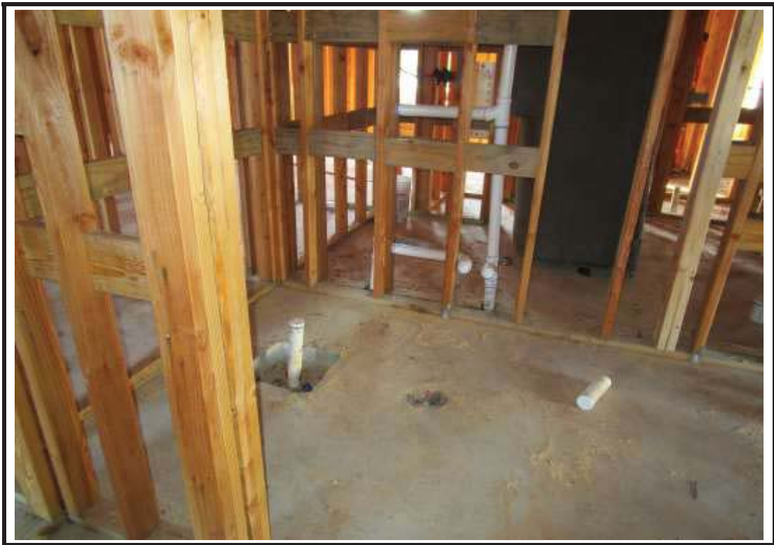
Photograph 5: Building 4 plumbing rough in.
