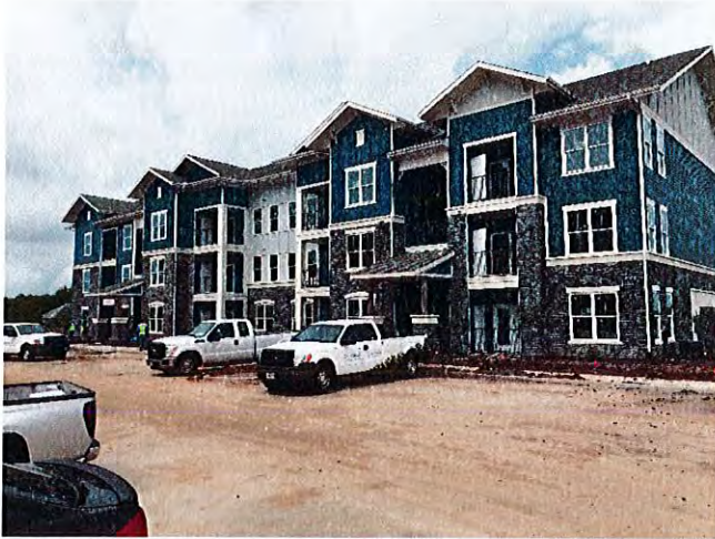
Overall view of building 4 with windows, siding and painting in place.
