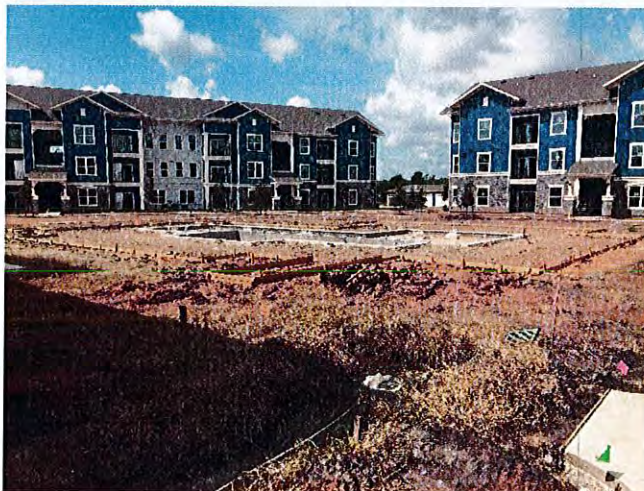
Overall view of the pool and on-going landscaping operations.
