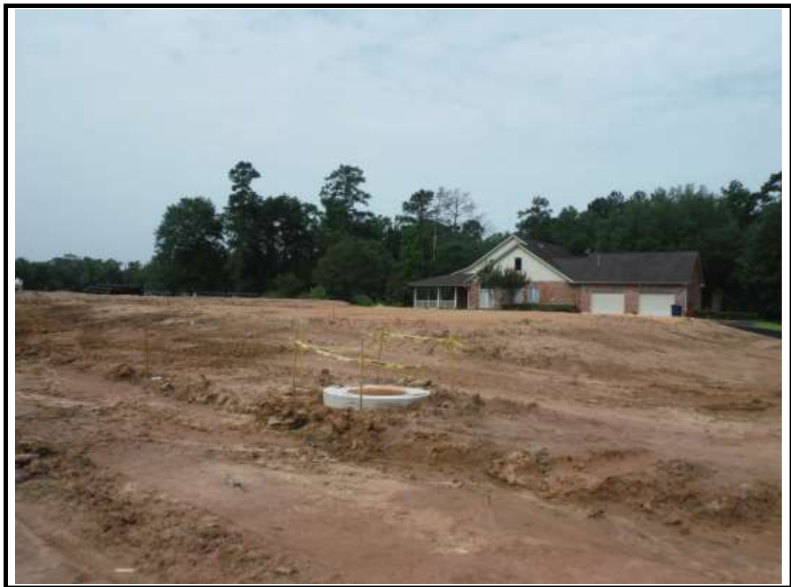
Photograph 14: Building 12 pad next to neighboring property.
