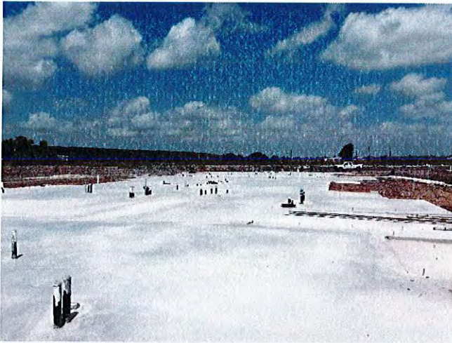
The slab at building 2 has been poured
