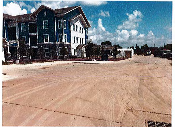
Landscaping was being installed around the buildings.
