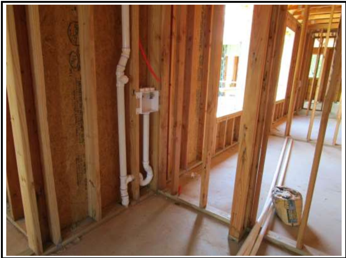
Photograph 3: Building 3 plumbing rough in complete.
