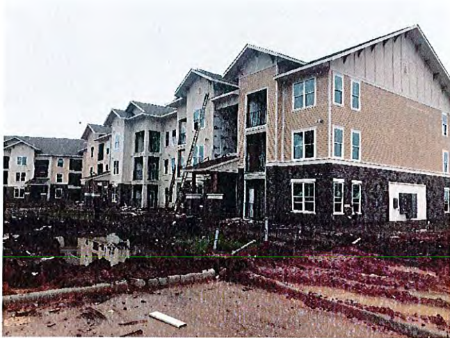
Overall view of Building #2 with siding substantially complete.
