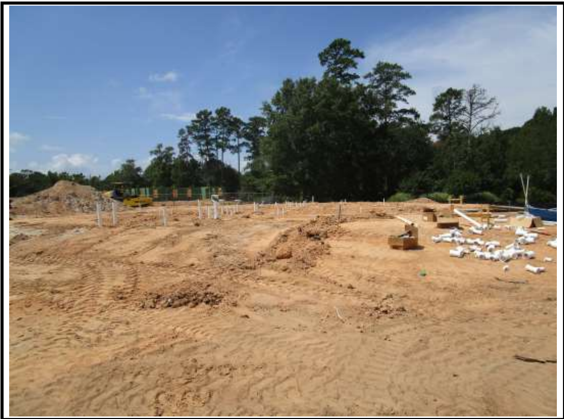
Photograph 14: Building 14 plumbing rough in underground in progress.
