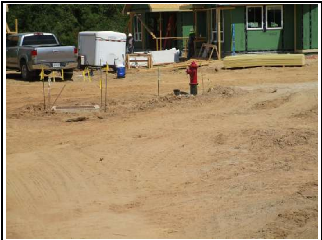
Photograph 7: Storm drain and hydrant by building 8.
