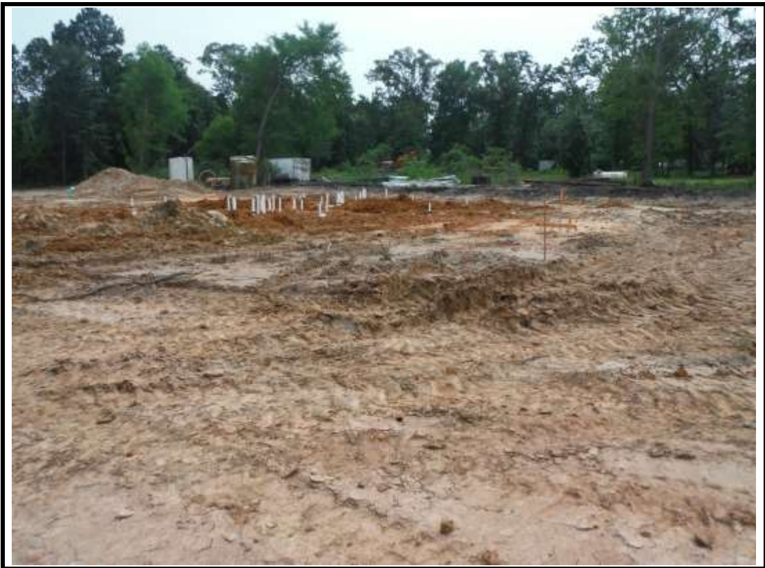
Photograph 10: Building 8 pad site.
