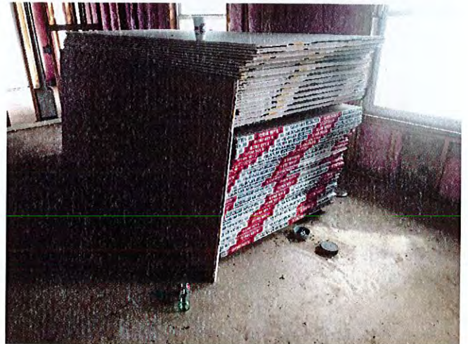
Drywall materials were being stockpiled inside the Clubhouse.
