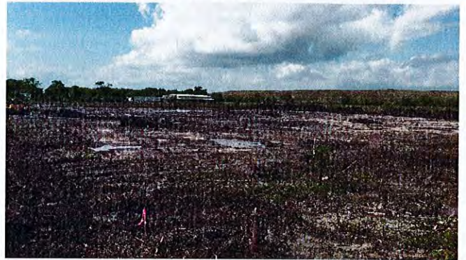
The site has been staked for cutting and filling.
