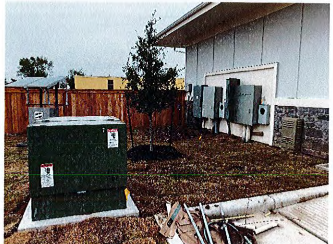
New power and electrical boxes had been installed.
