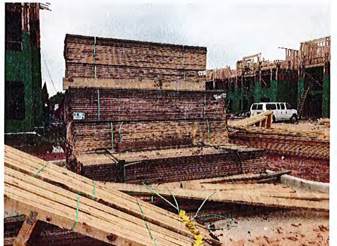
Rough framing materials were being stockpiled on site.
