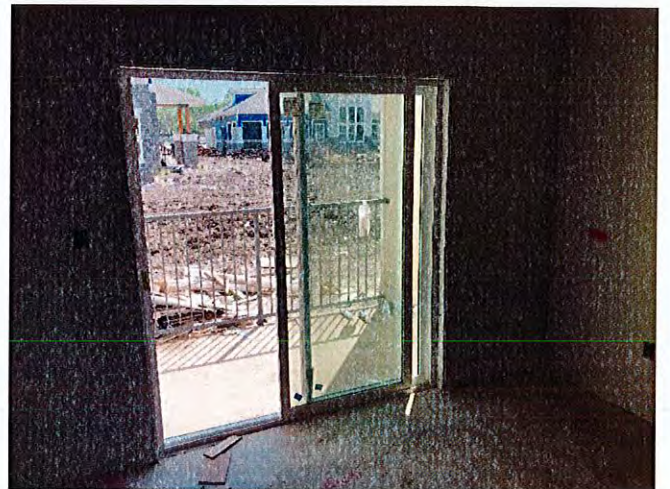
Sliding glass doors were in place at building 2.
