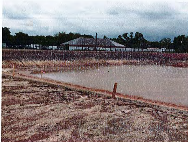
Excavation of the detention pond is underway.
