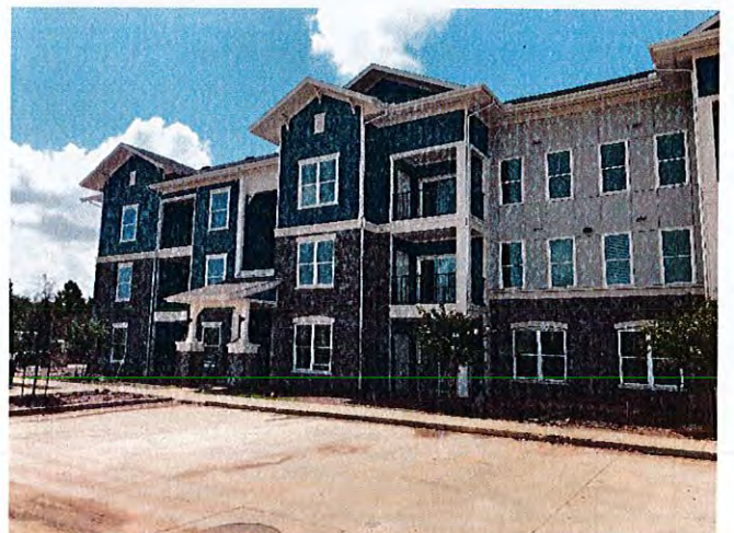
Overall view of building 1 with landscaping operations underway.
