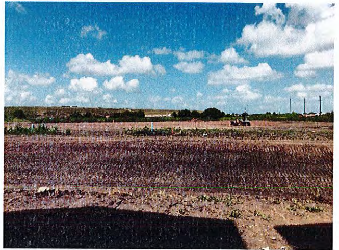
Overall view of the cricket field which had earthwork substantially complete.
