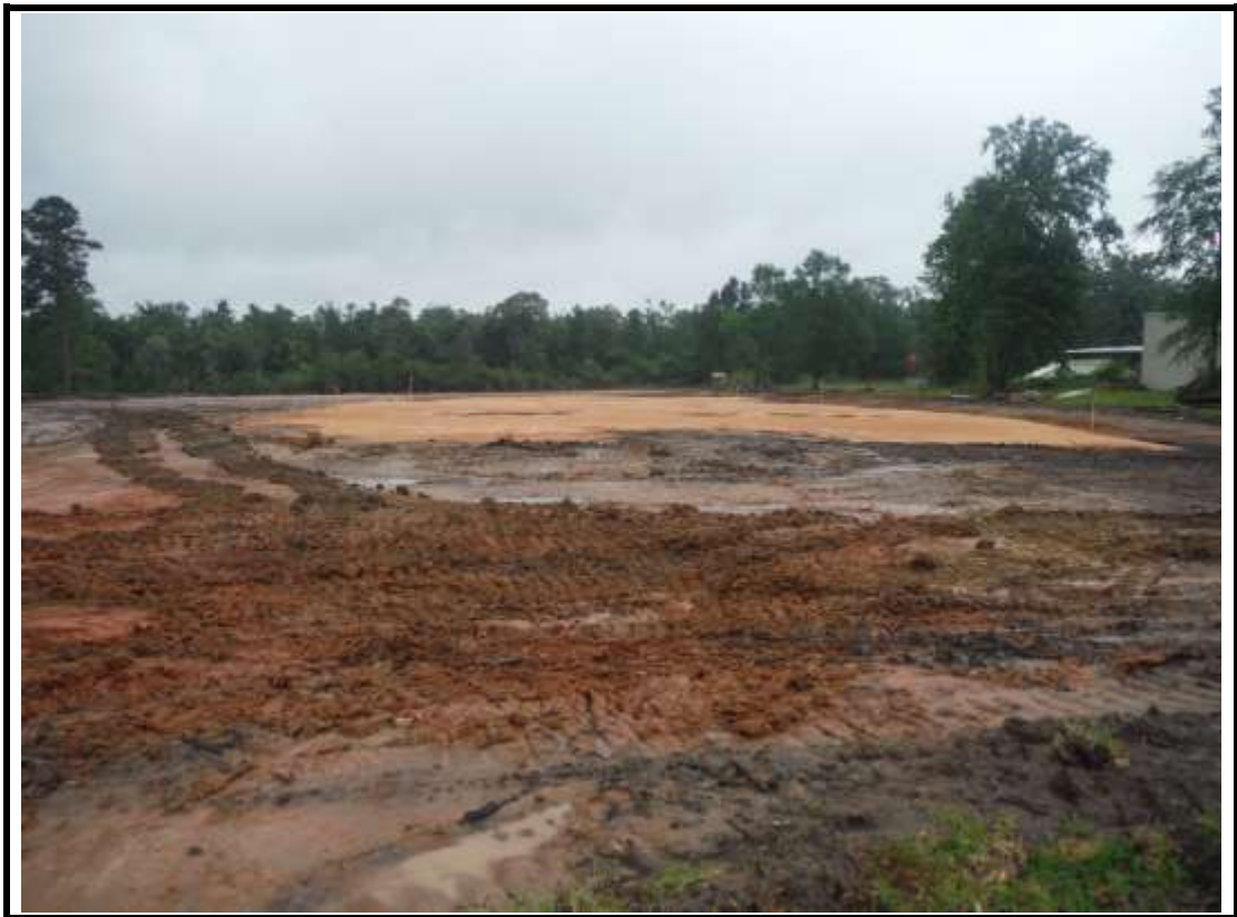
Photograph 4: Site work facing Building 1 pad.
