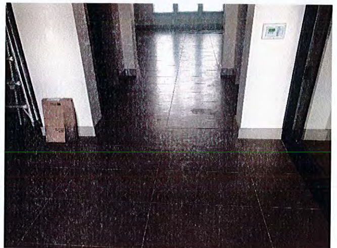
Floors had been installed at the clubhouse.
