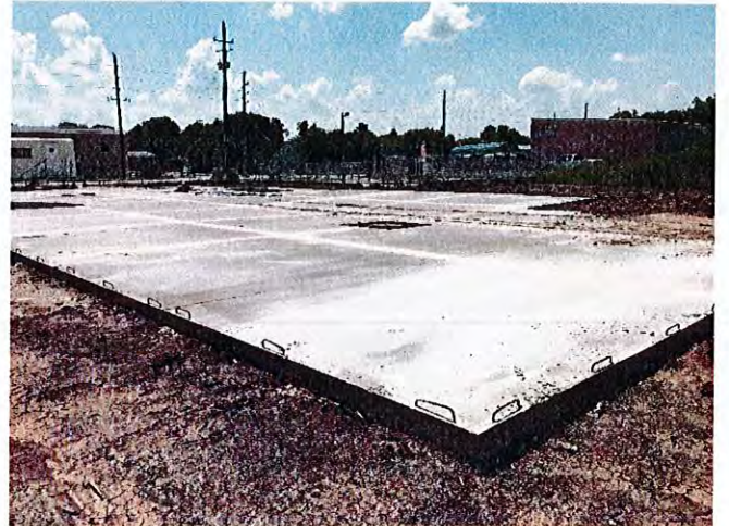
Overall view of a portion of the completed paving areas.
