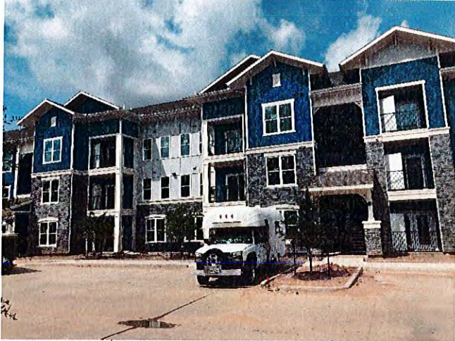
Overall view of building 3.
