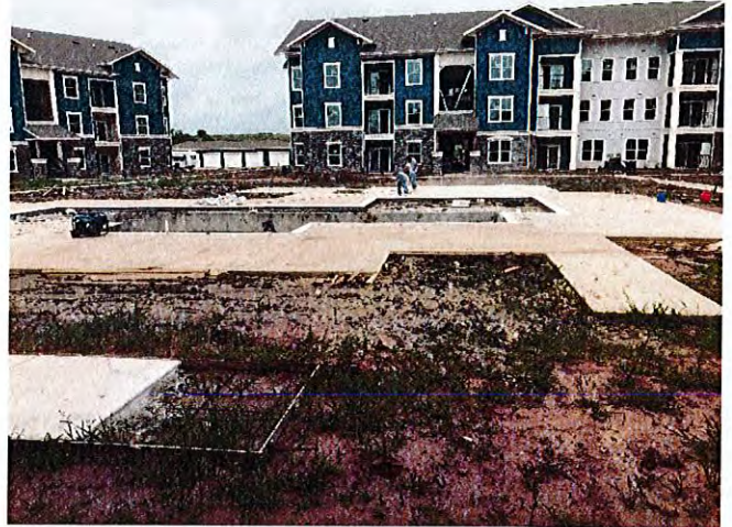
Overall view of the courtyard with the pool nearing completion.
