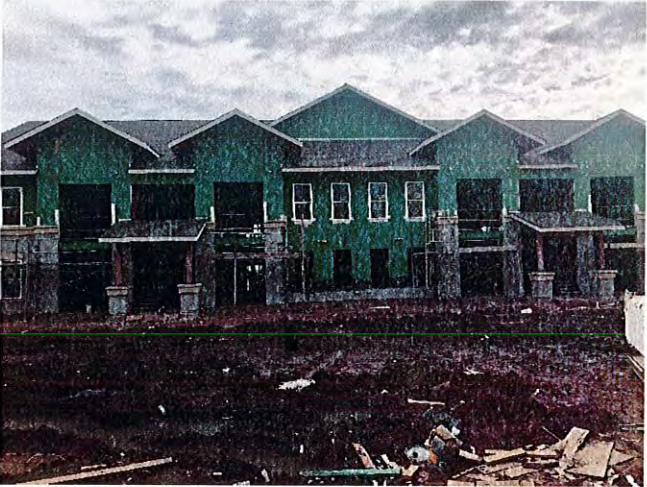
Siding was being installed on the south end of Building #6.
