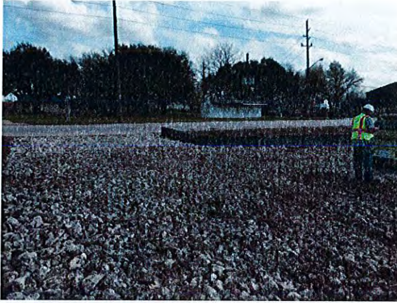
1. Rip rap construction entrance.
