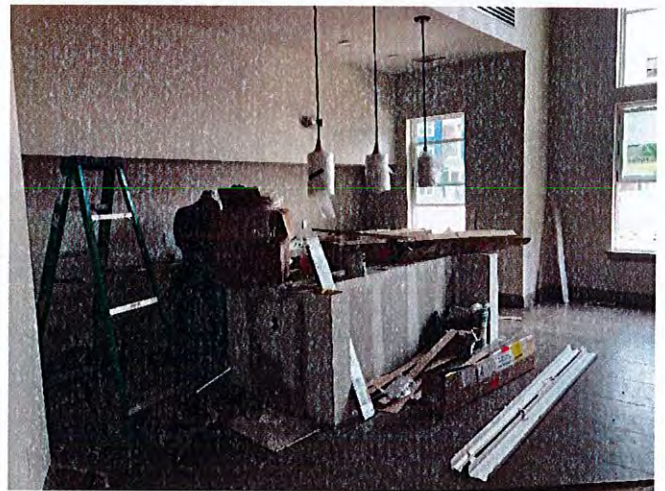
Drywall was nearing completion and painting operations were underway.
