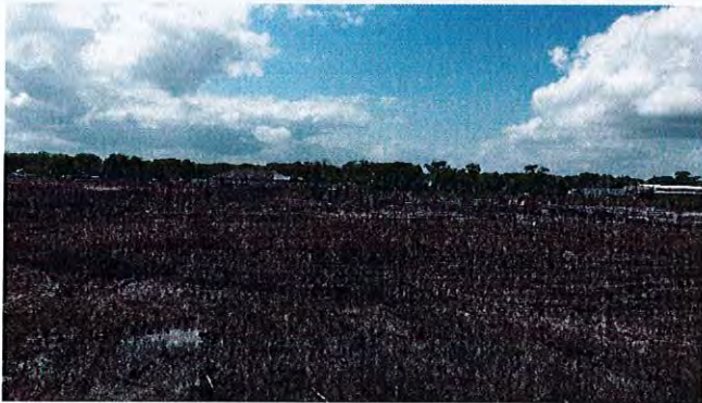
The excavation of building pad #2 is underway.
