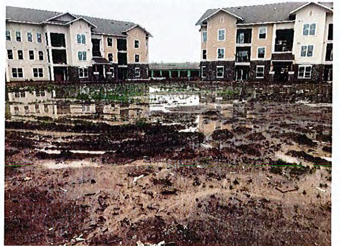
Overall view of the jobsite conditions.
