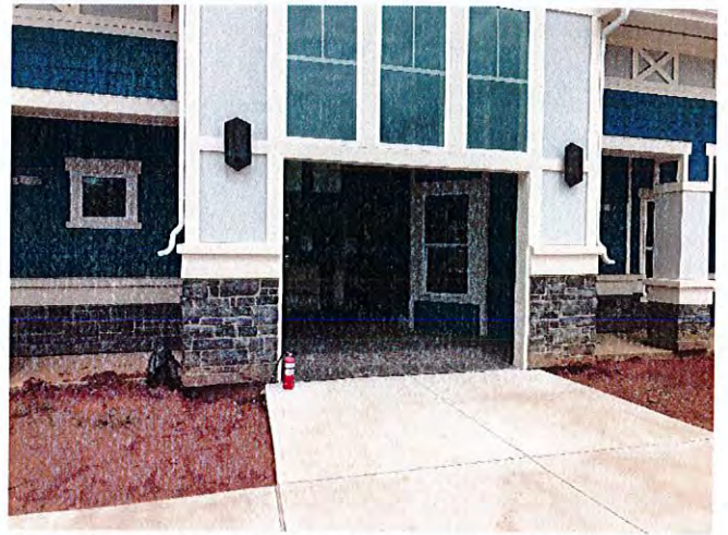
Storefront of the clubhouse was nearing completion.
