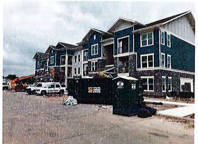
Overall view of building 4 with painting upgrades substantially complete.
