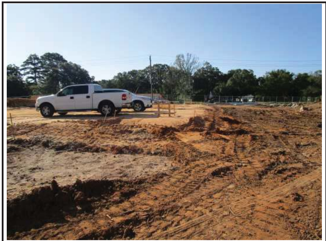
Photograph 16: Building 19 pad progress.
