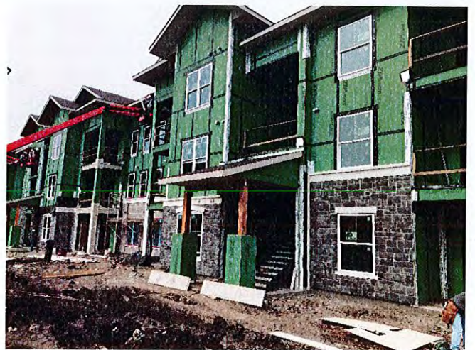
Overall view of Building 1.
