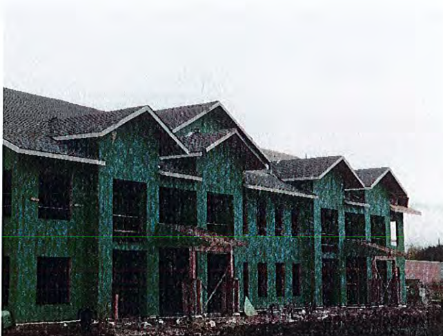
Overall view of building 4.
