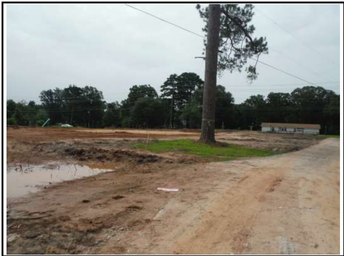
Photograph 16: Building 18 pad site.
