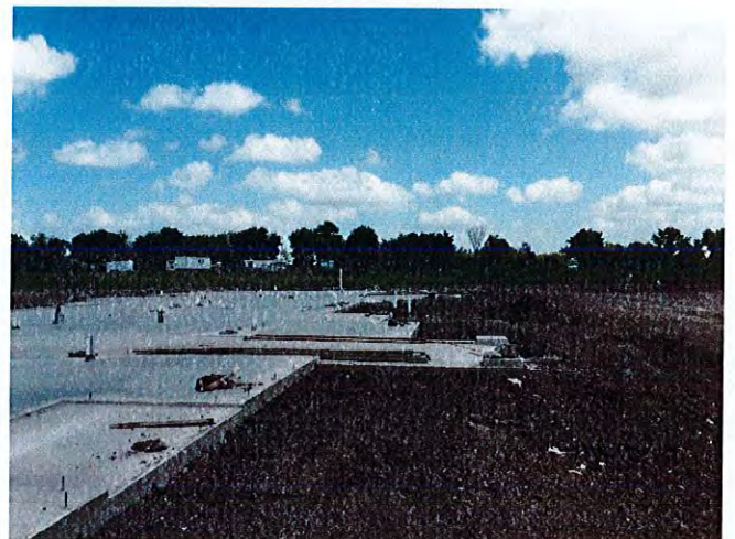
The slab at building 3 has been poured.
