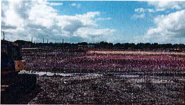
The pad at the clubhouse is in progress.
