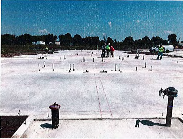
Overall view of Building 1 slab.
