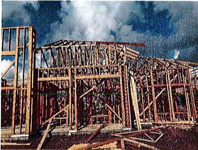
Rough framing operations are well underway on the club house.
