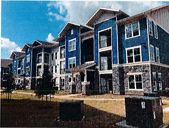
Overall view of building 2 with exterior work substantially complete.
