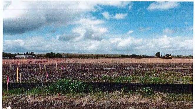
In the background the detention pond excavation is nearing completion.
