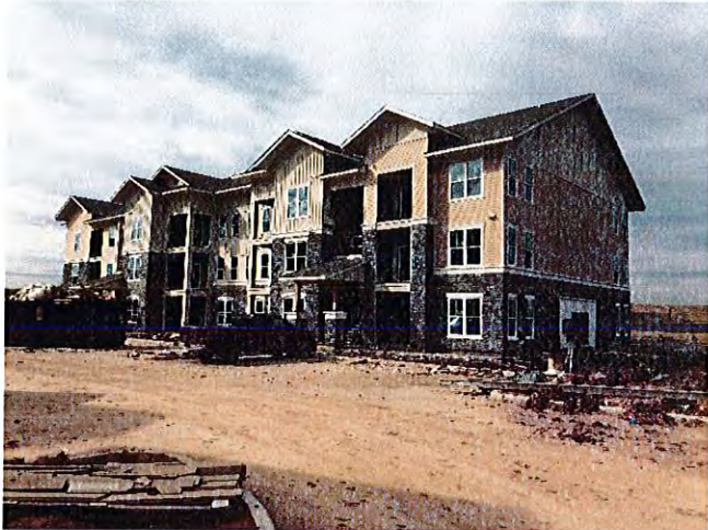
Overall view of Building #4.
