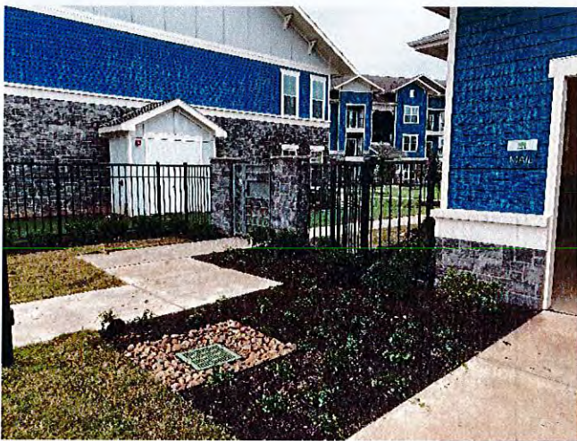
Landscaping was nearing completion around the job site. Gates around the club house had been installed.
