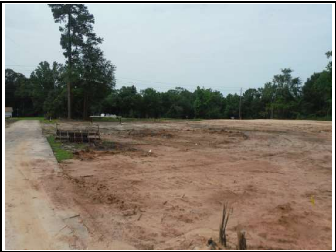
Photograph 15: Pad site building 14.
