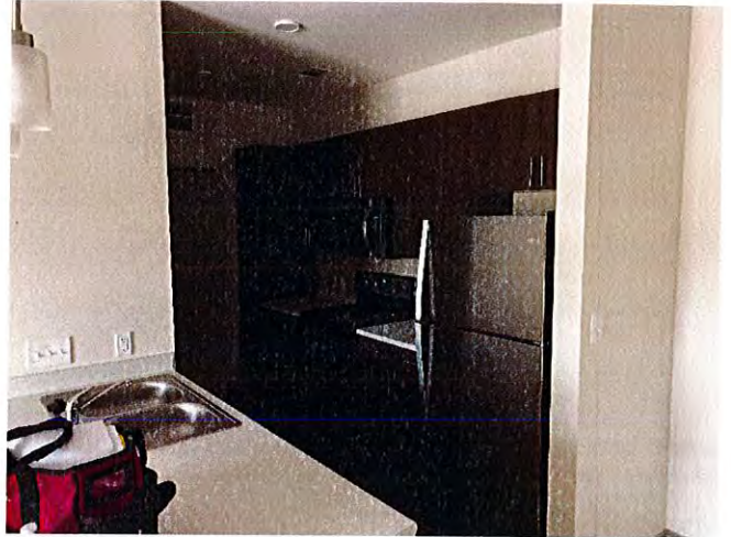
Appliances had been installed at unit 1201.
