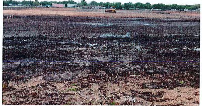
Select fill has been added at building pad #1.
