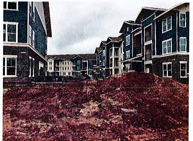
View of conditions in the courtyard.
