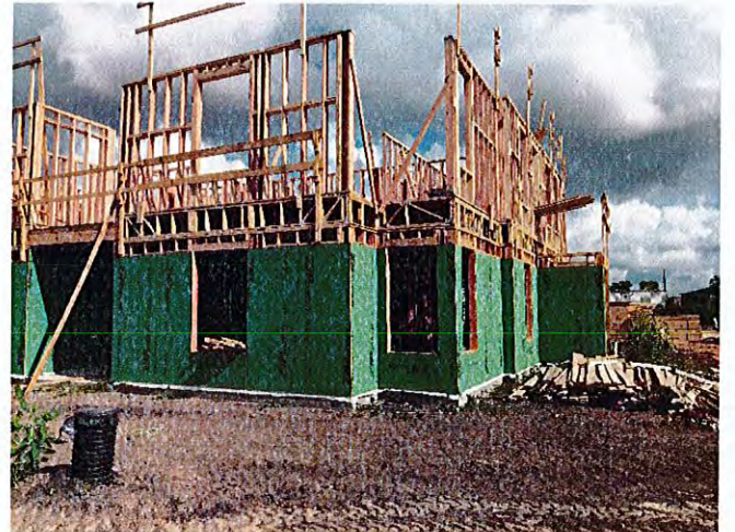
Rough framing on the second floor is underway on Building 1.
