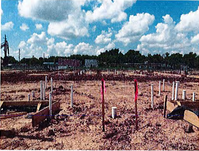
Underground utilities, staking and formwork is underway at building #3.
