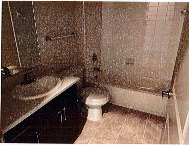
The bathrooms were substantially complete at building 1.
