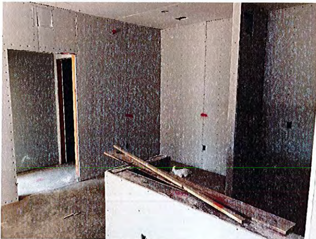
Interior drywall operations were well underway at building 2.
