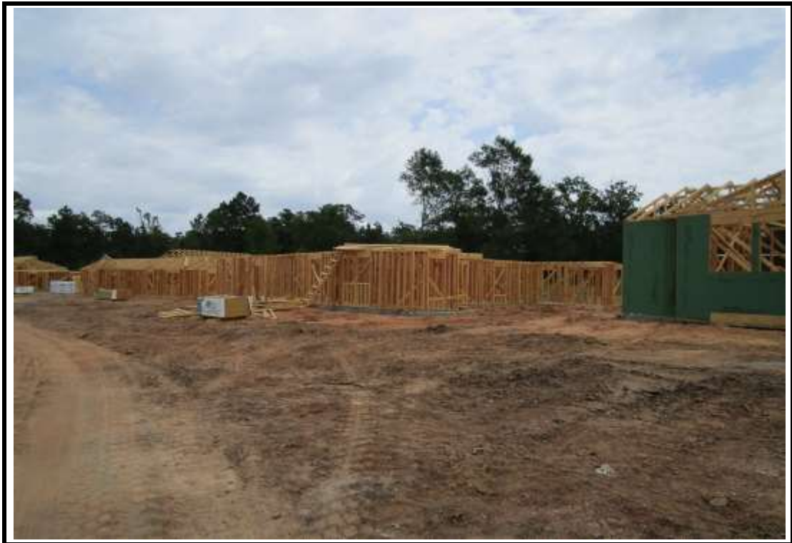
Photograph 6: Building 8 framing in progress.
