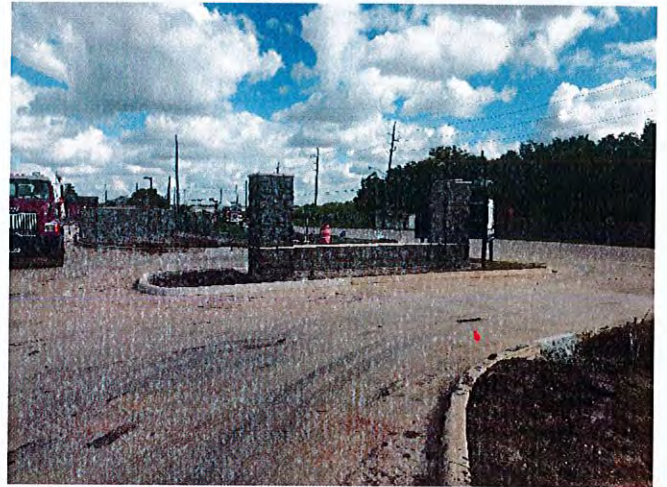
Masonry work for the signage was in place.
