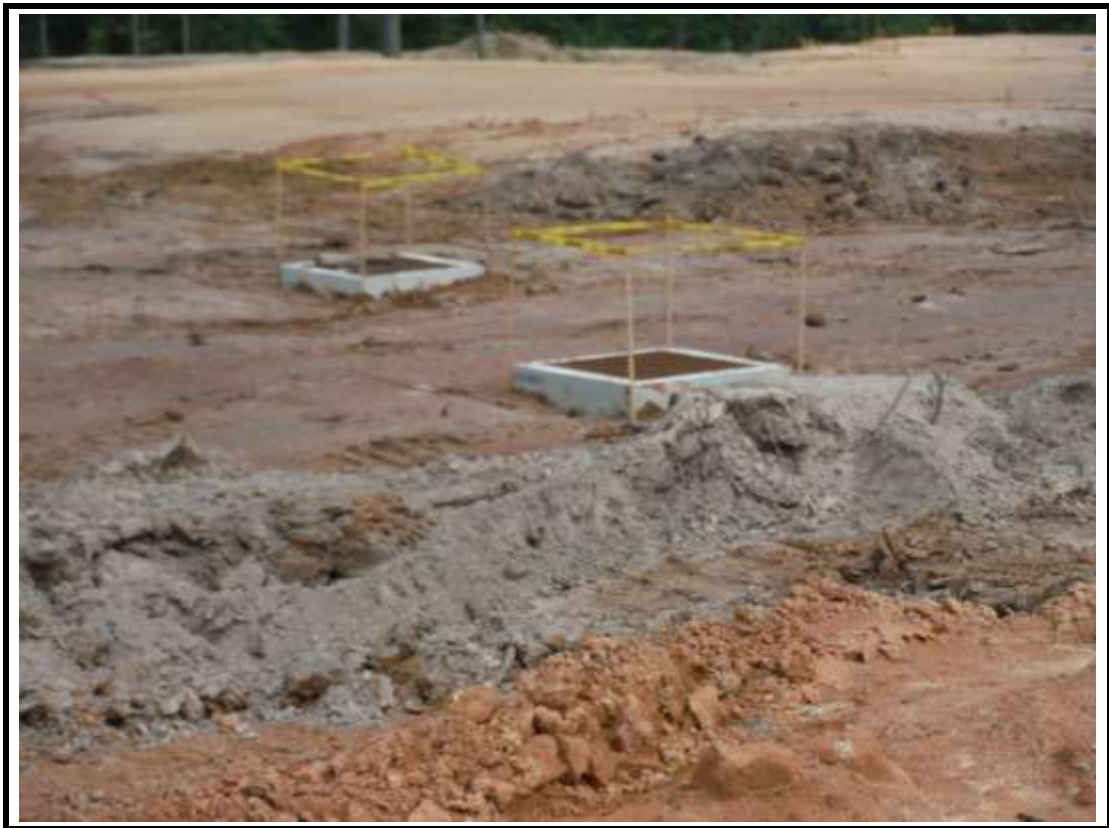
Photograph 7: Street storm sewer vaults.
