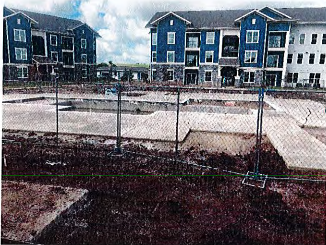
Concrete around the pool appeared to be in place.
