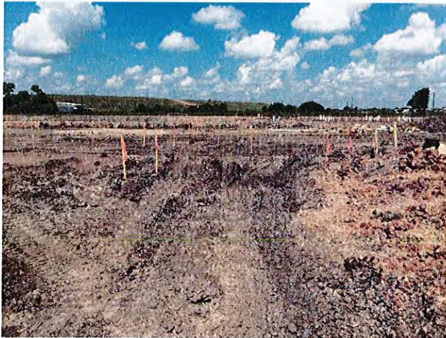
Staking throughout the site is nearing completion.
