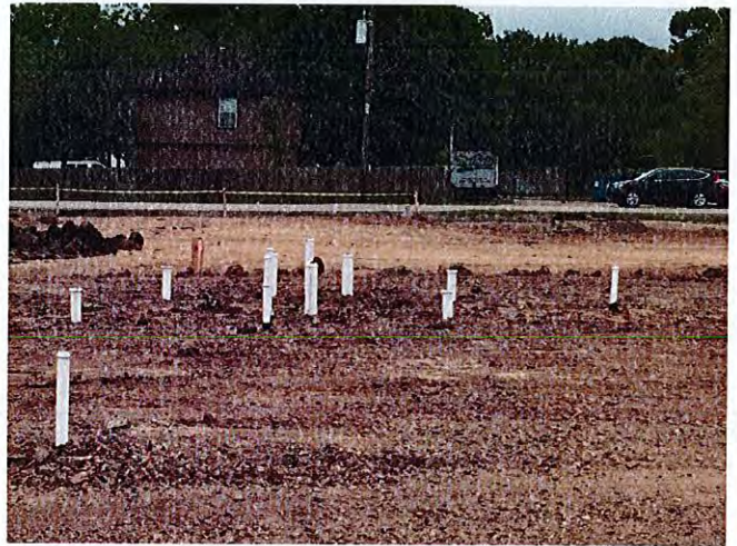
Stubbed up plumbing at a portion of building 1.
