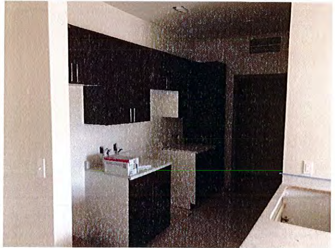
The cabinets had been installed in the kitchen.
