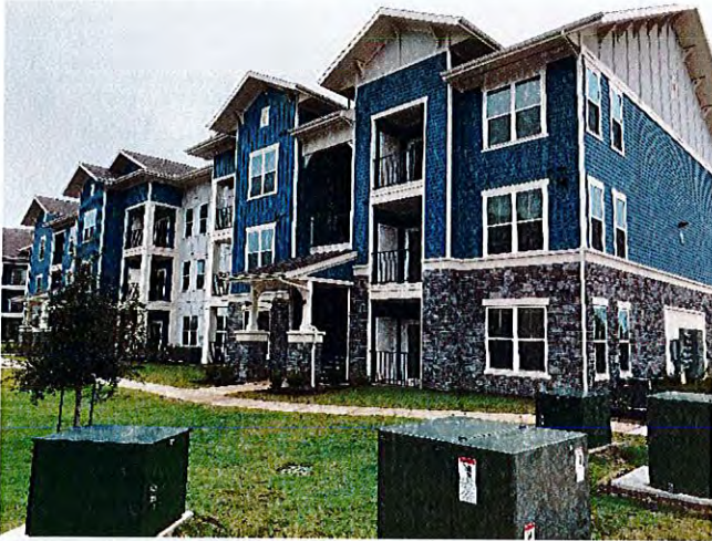
View of building 1 which is substantially complete.
