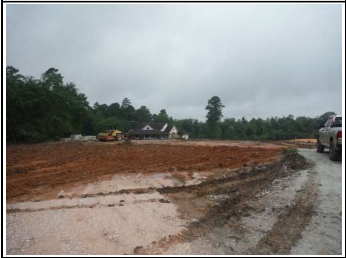
Photograph 3: Site work towards neighboring house.
