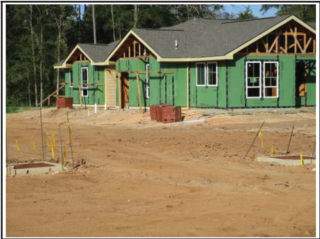
Photograph 9: Building 10 roofing complete.
