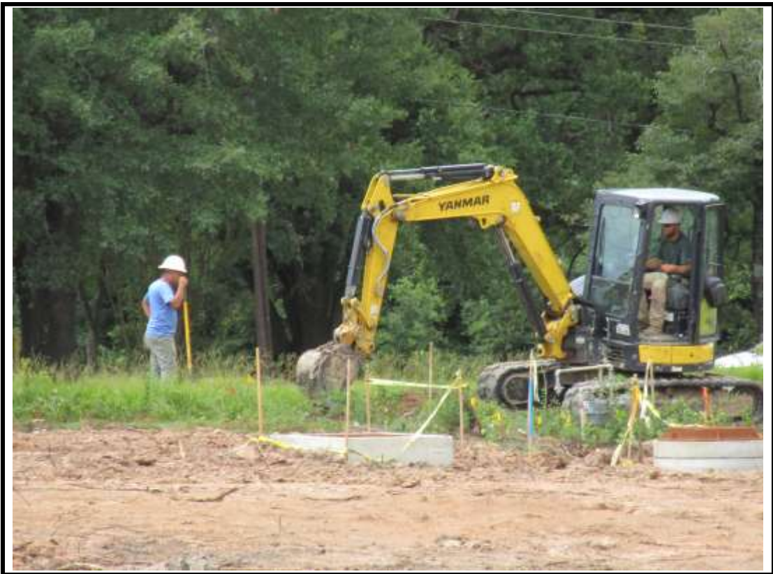
Photograph 16: Water line relocation in progress along front of property.
