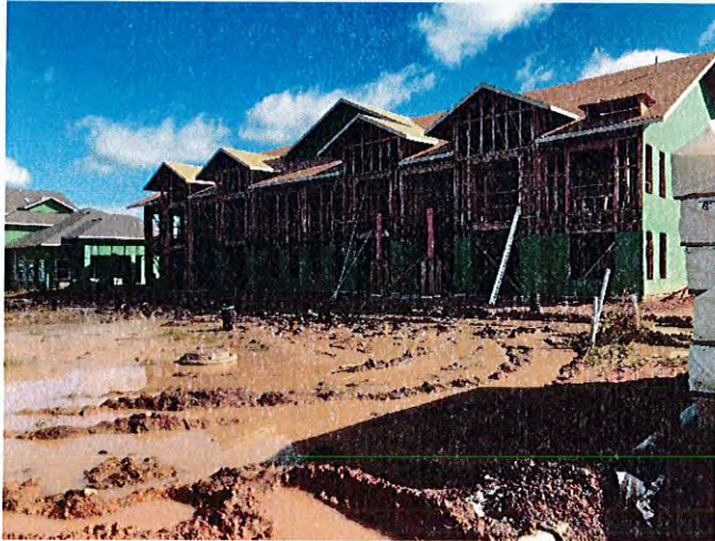
Overall view of building 4.
