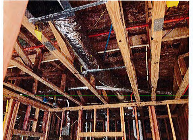
HVAC ductwork was being placed in building 1.
