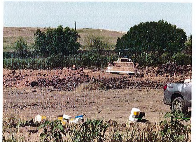
Excavation work was underway at the cricket field.
