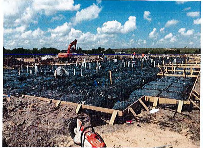
The formwork and vapor barrier are substantially complete at building #1.
