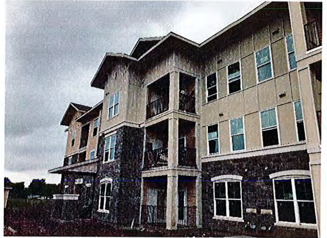
Overall view of building 4 with painting upgrades underway.
