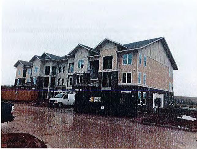
Overall view of Building #3 with siding nearing completion.
