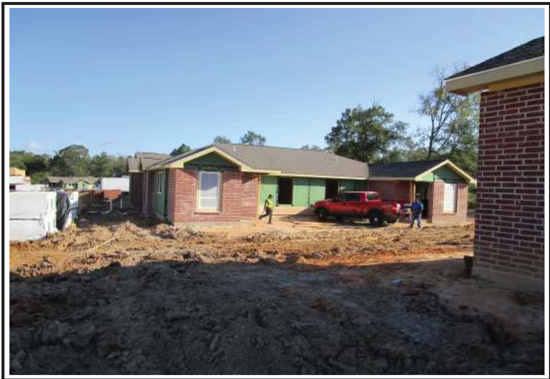
Photograph 6: Building 5 exterior progress.
