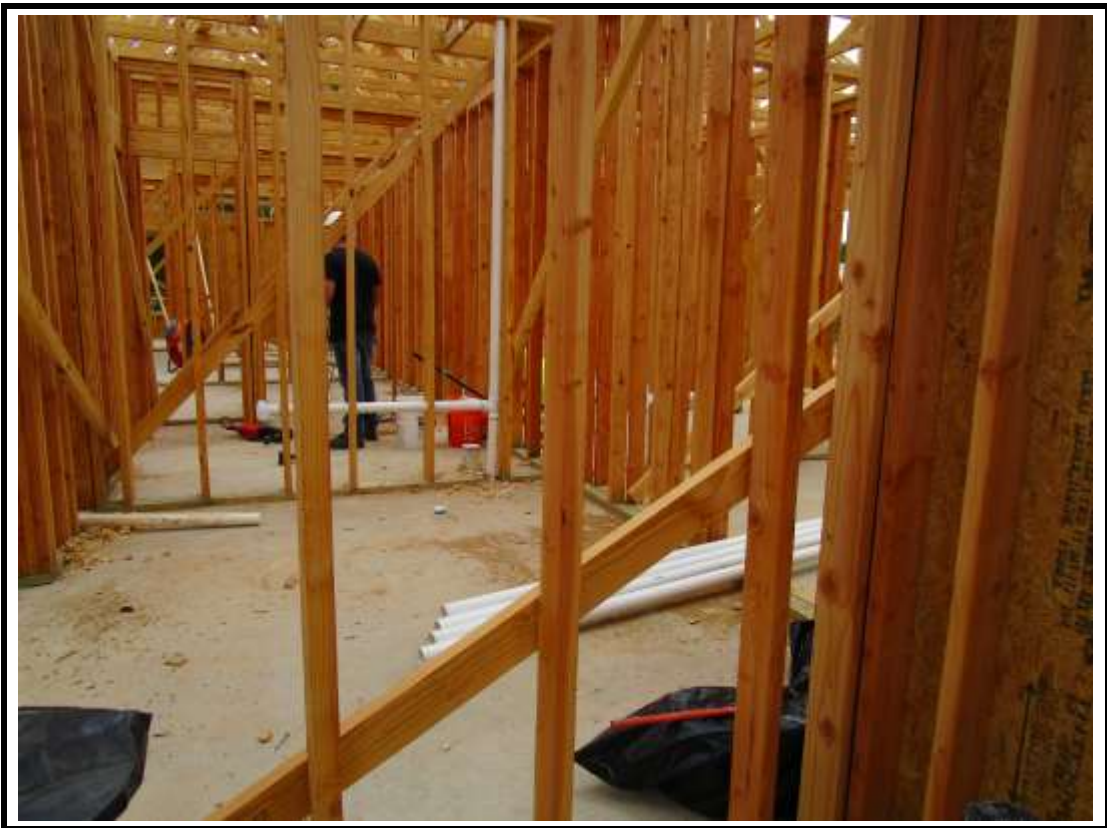
Photograph 3: Building 1 plumbing rough in progress.
