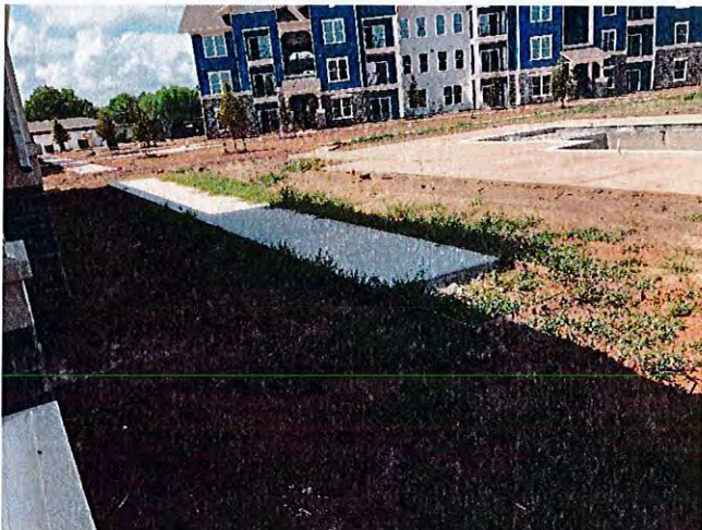
Sidewalks were being poured at the south end of the clubhouse.
