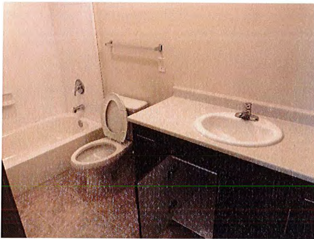
Unit 3104 had the bathroom nearing completion.
