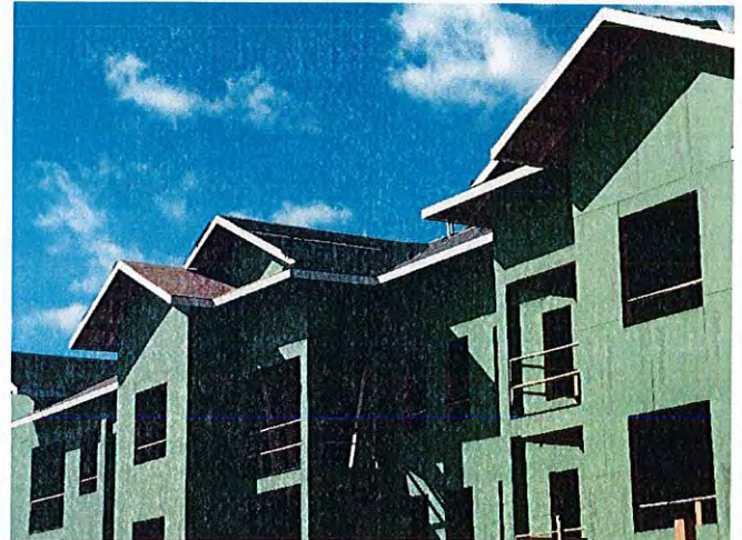
Roof was substantially complete on building 2.
