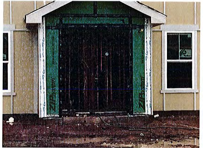
Electrical and plumbing was substantially complete at building 4.
