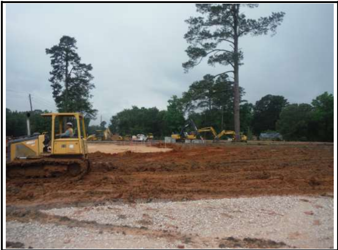
Photograph 2: Site & pad work on Clubhouse.
