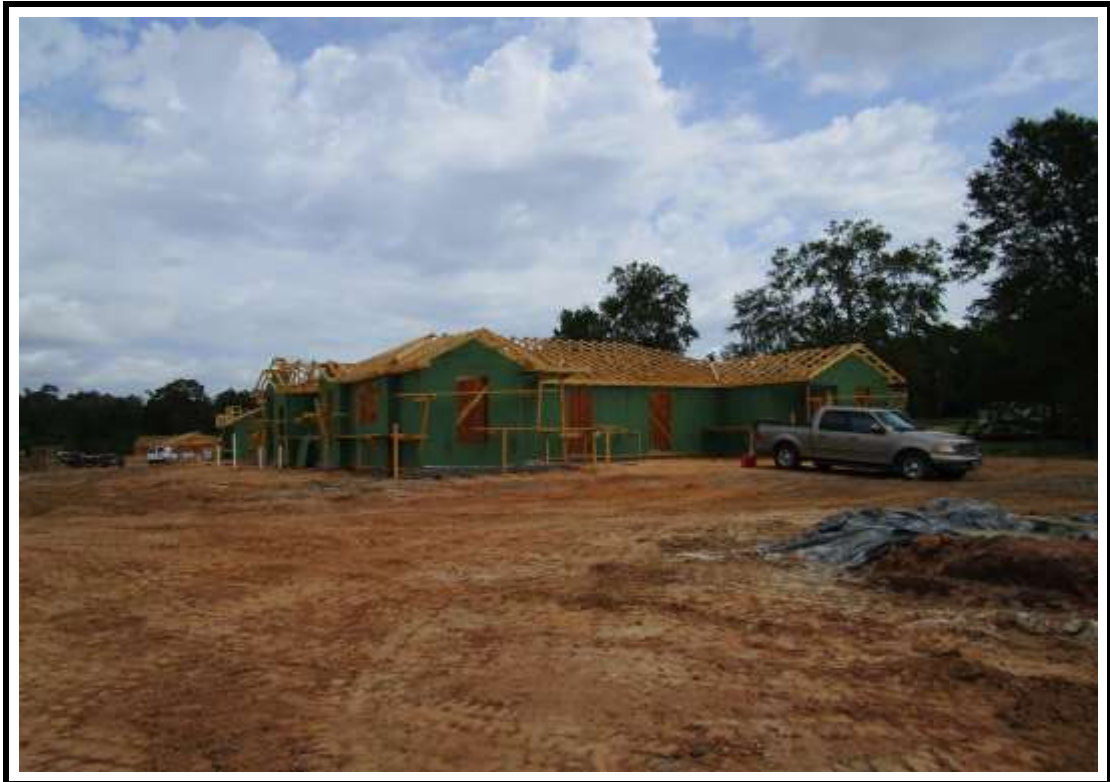
Photograph 2: Building 1 framing complete.
