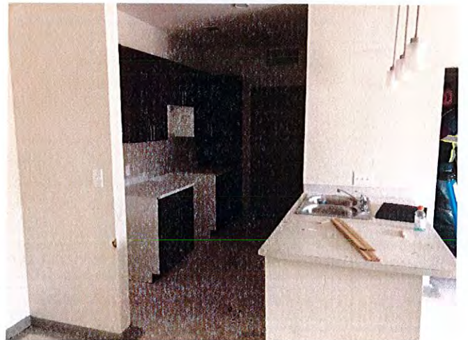
View of a kitchen in a unit at building 2 with countertops and cabinets in place.
