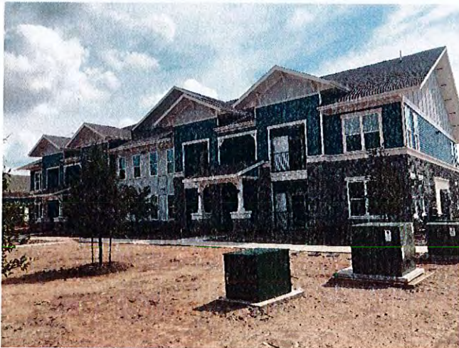
Overall view of building 6.
