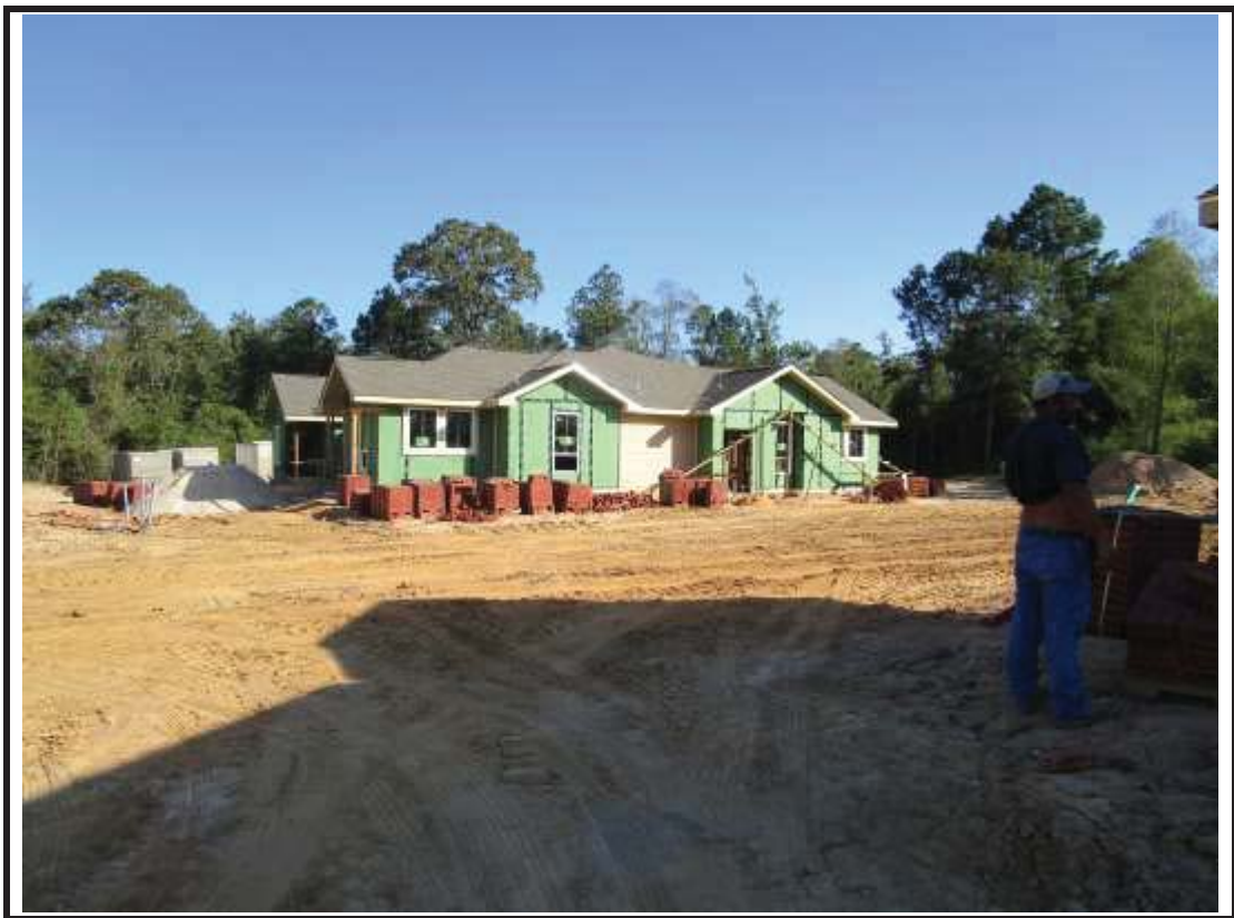
Photograph 8: Building 8 exterior brick installation beginning.
