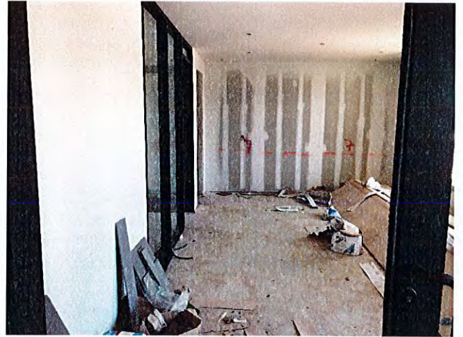
Interior drywall was nearing completion.
