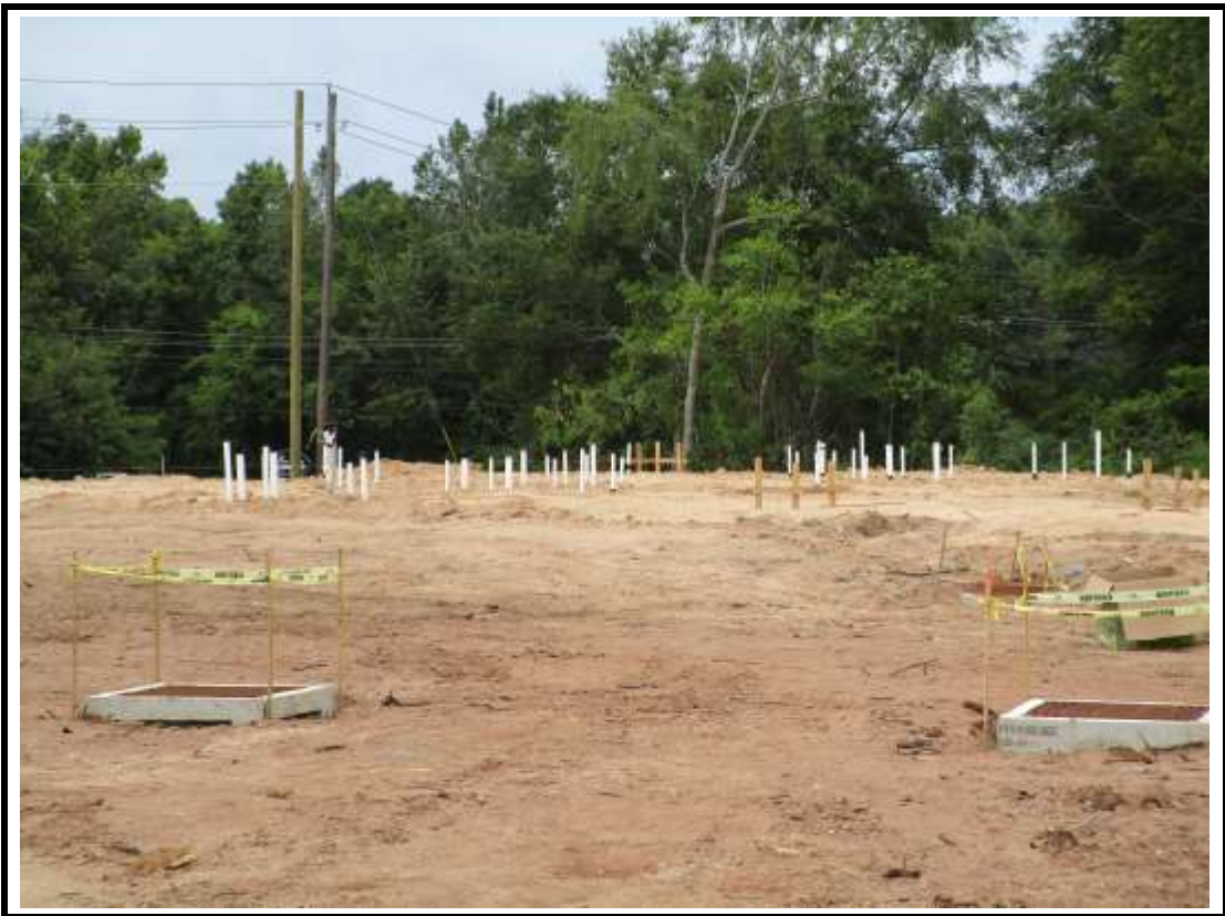
Photograph 15: Pad site building 17, plumbing underground.
