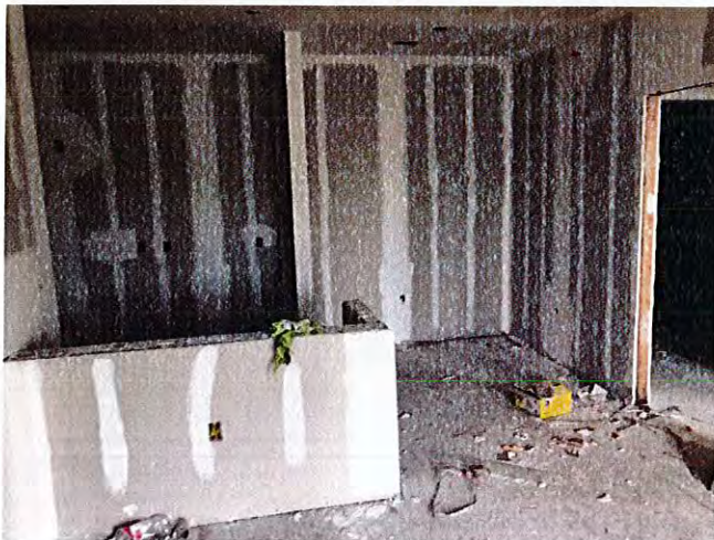
Drywall was substantially complete throughout building 4.
