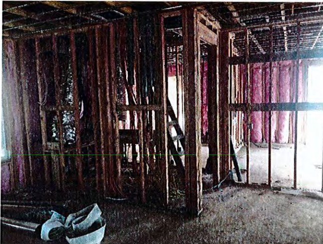
HVAC and electrical work was well underway at the Clubhouse.
