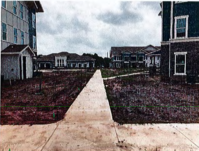
Concrete sidewalks had been installed throughout the job site.
