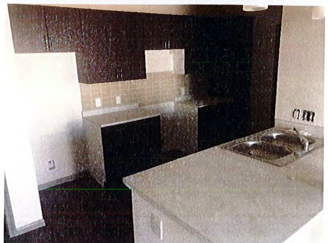
Unit 5103 was awaiting installation of appliances.
