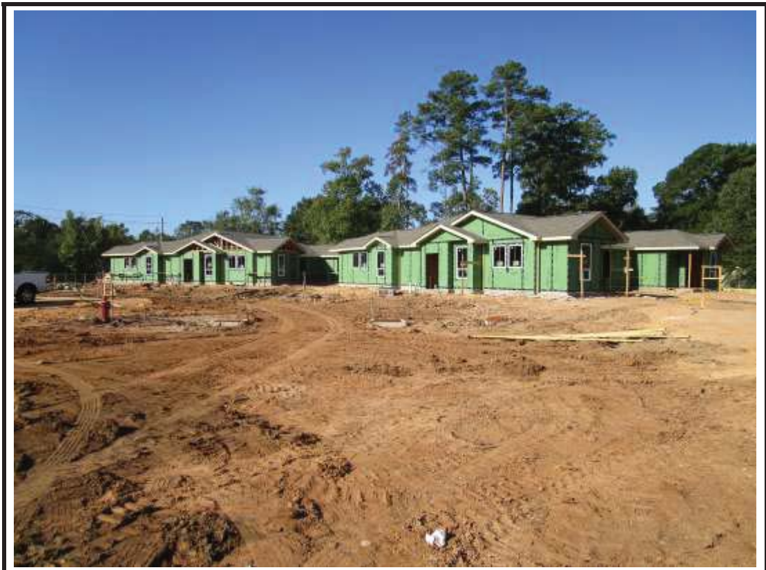
Photograph 11: Buildings 9 & 10 exterior progress.
