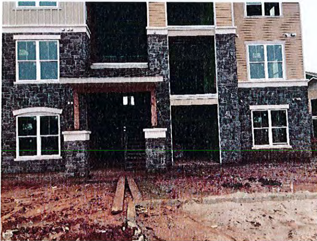
Masonry operations were nearing completion at building 6.
