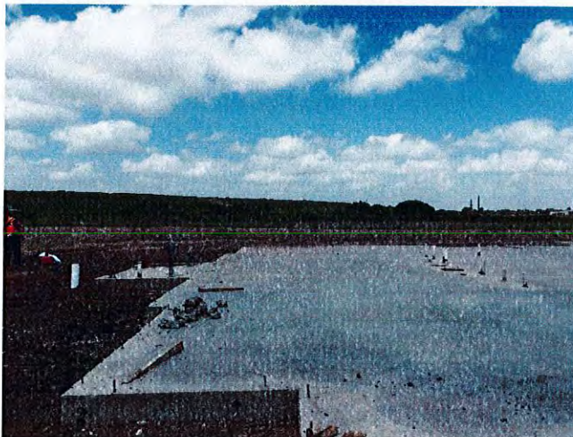
The slab at building 4 has been poured.
