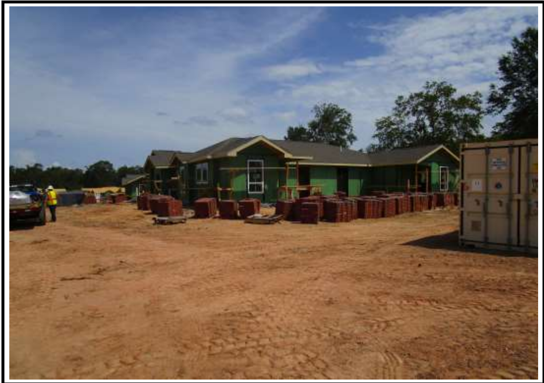
Photograph 2: Building 3 roof completed.
