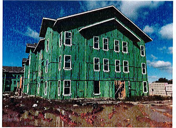
Overall view of building 1.
