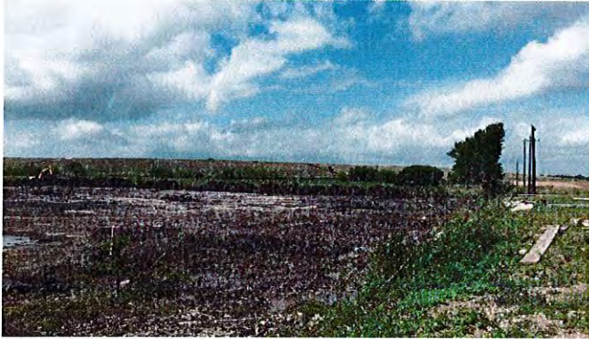
Rough grading at building pad #4 is underway.
