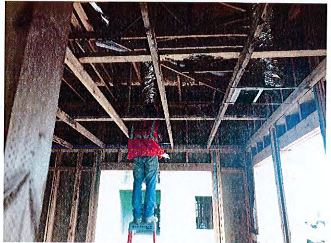
HVAC ductwork was being installed at the Clubhouse.
