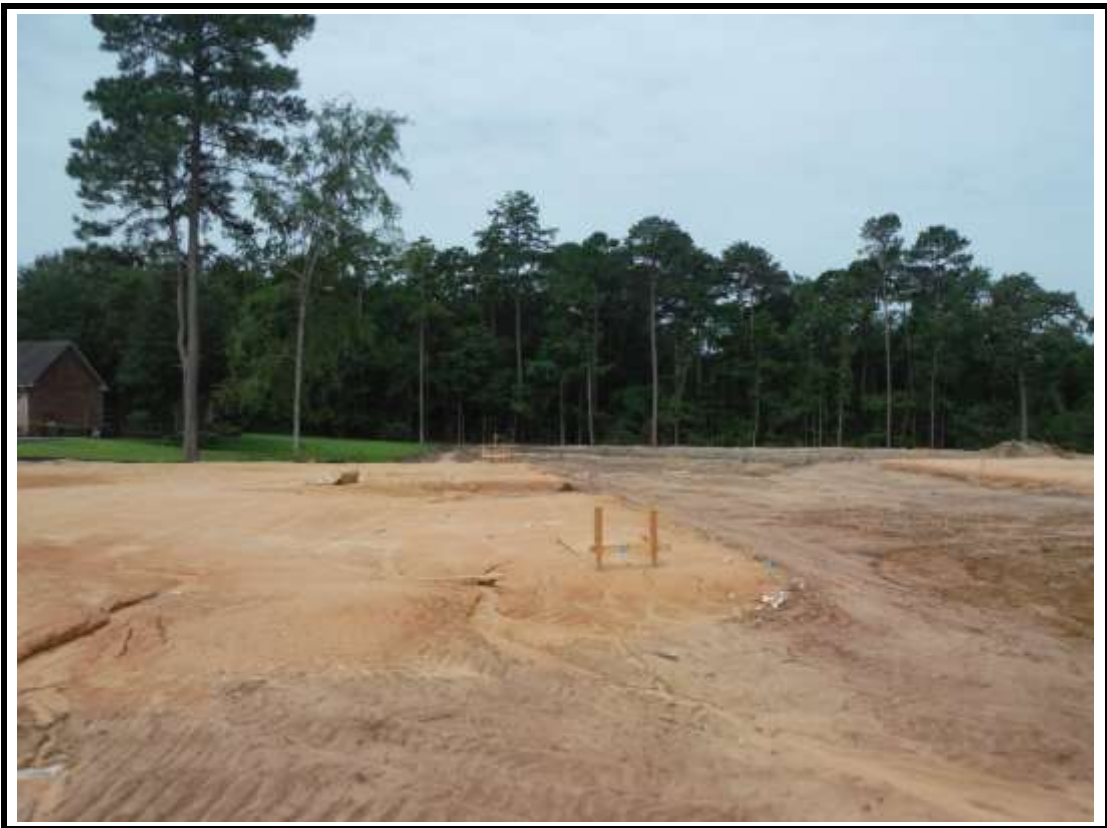
Photograph 13: Detention pond site at end of drive.
