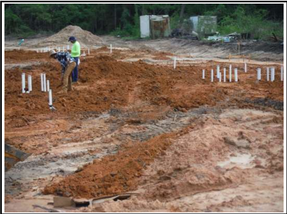
Photograph 9: Building 7 pad site plumbing rough in.
