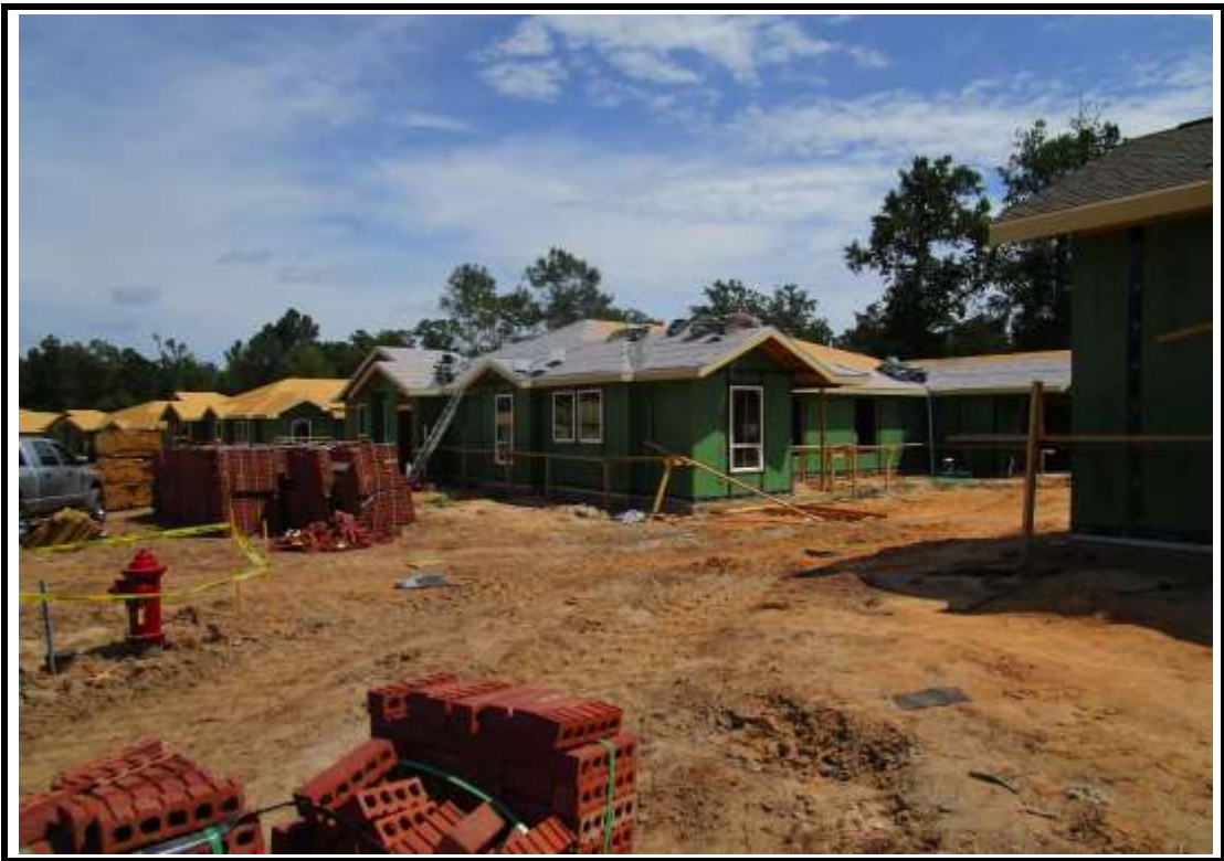
Photograph 5: Building 5 & 6 roofing in progress.
