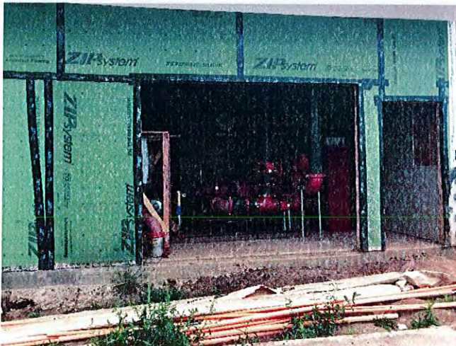
Installation of the fire sprinkler system was well underway.
