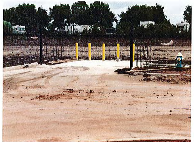
The concrete pad for the trash enclosure was substantially complete.
