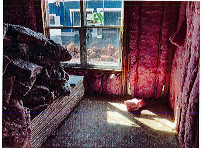
Interior windows had been installed and insulation was nearing completion.
