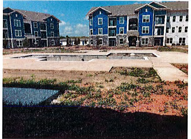
Overall view of the courtyard with the pool nearing completion.
