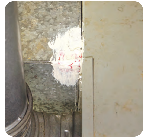
B-3. Apply mastic over the tape
