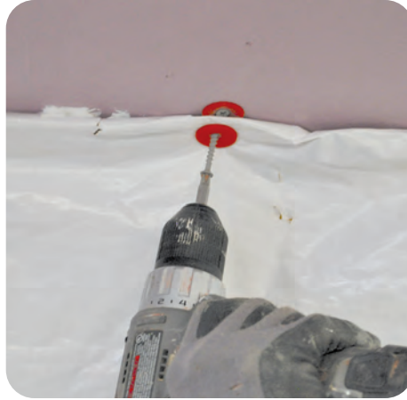
2. Attach new belly wrap
