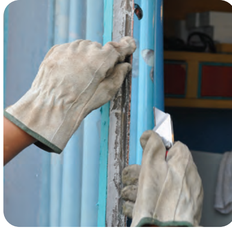
2. Clean all debris, caulk, etc., from sash
