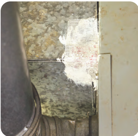
B-4. Push fiberglass mesh into the mastic
