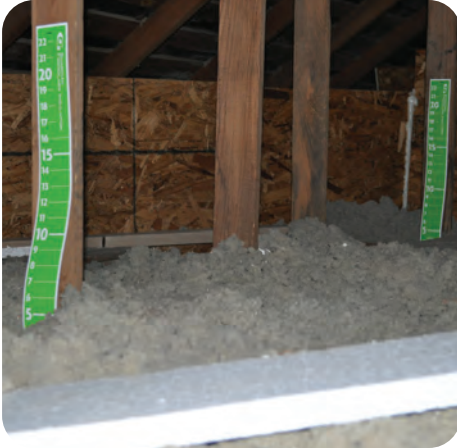
5. Depth rulers installed, 1 per 300 square feet
