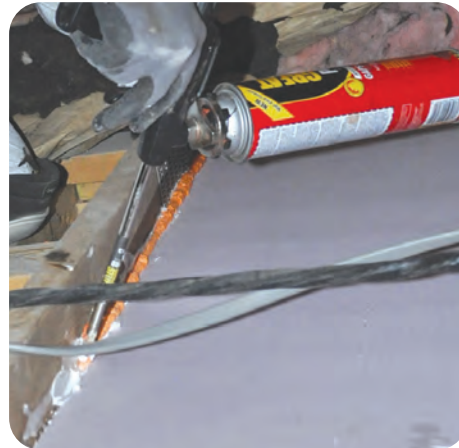
B-2. Seal around infill materials
