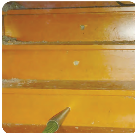
11. If backside of stairs is already sealed, blow insulation into cavity behind stairs
