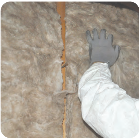
3. Install batts with minimal compression
