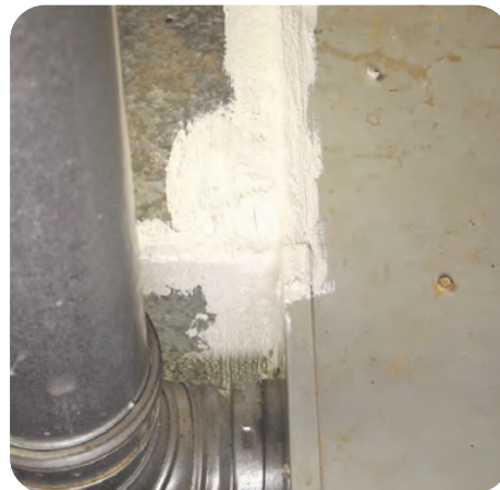
B-5. Apply additional mastic over mesh and tape, extending at least 1 inch past edges of tape in all directions
