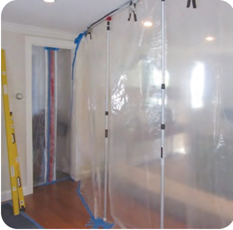
1. Protect work area from debris and dust
