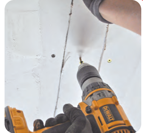
7. Fill and reseal access holes to prevent air movement
