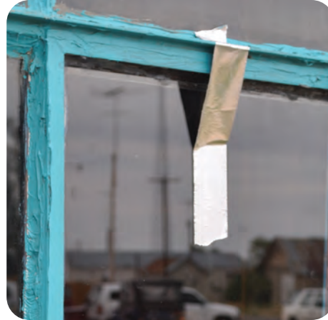
6. Hold new pane with tape or stops
