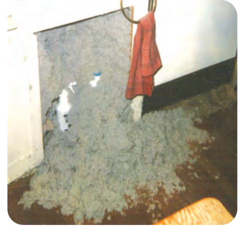
3. Ensure wall integrity is complete (no holes)
