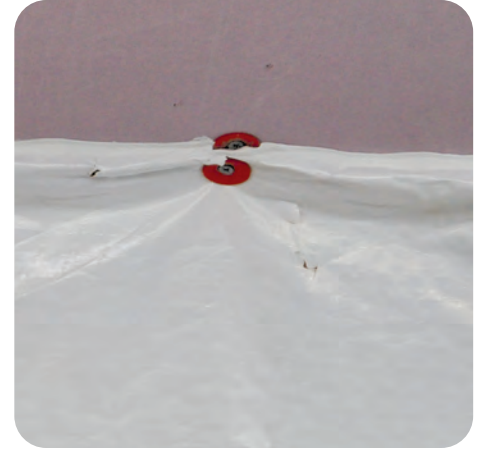
3. Seal seams of belly wrap
