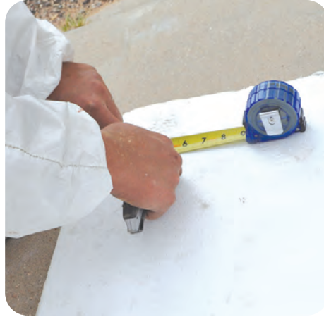
2. Cut blocking material to fit
