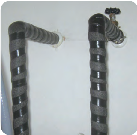
Secure seams with tape
