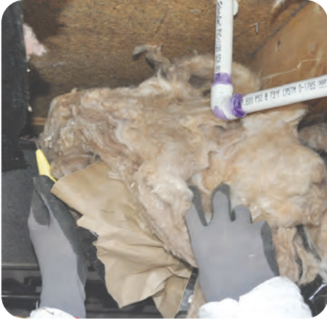
1. Remove old insulation and make repairs as needed
