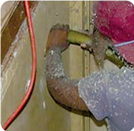
7. Dense pack stairway walls
