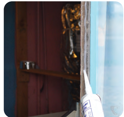
4. Run interior bead of caulk
