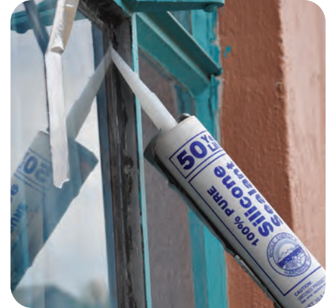
7. Caulk all edges
