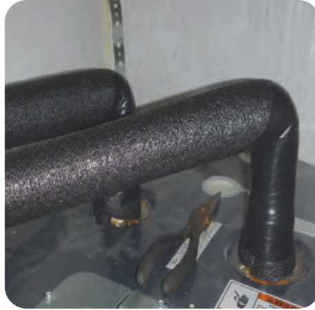
Insulation should be continuous with no gaps, corners mitered and secured
