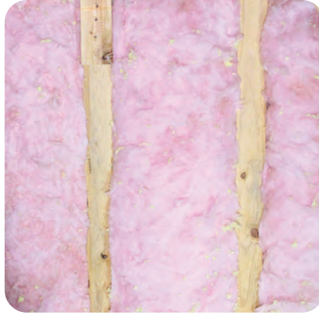
2. Cut batts for exact fit
