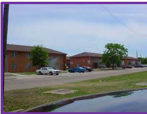
Carver Terrace/Lincoln Square Apartments in Port Arthur, Texas.
