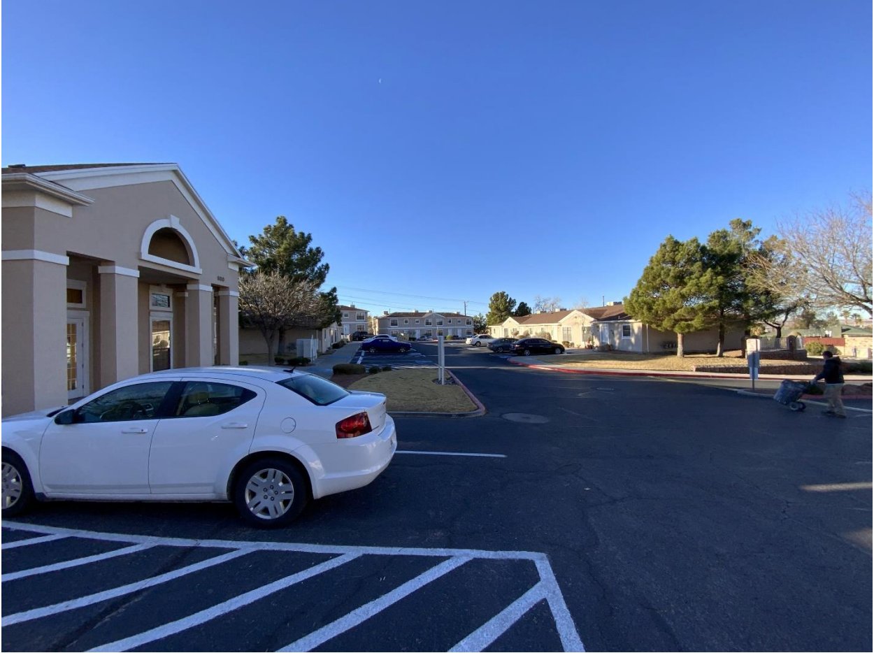
Clubhouse, Building 1 and 2 parking area
